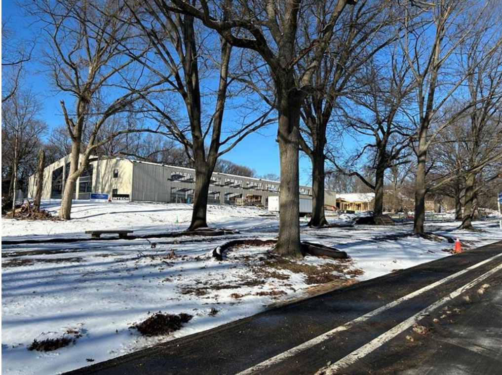
Entire building facade
