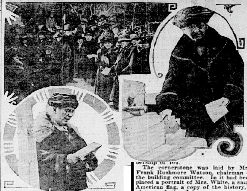
Members of the Woman's Club of Germantown yesterday afternoon laid the cornerstone of their new house at Germantown avenue and Washington lane. A group of the participants is shown above at left while at right Mrs. Frank Rushmore Watson is laying the stone in place. Below Mrs. Walter Penn Shipley is delivering the dedicatory address.
