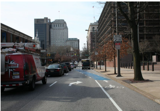
Colored pavement (4.5.11) can be used to increase visibility of potential bicycle/vehicle conflict zones. Green color must be used for all future applications.
