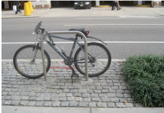
Different materials may be used to differentiate the furnishing zone and allow stormwater infiltration.
