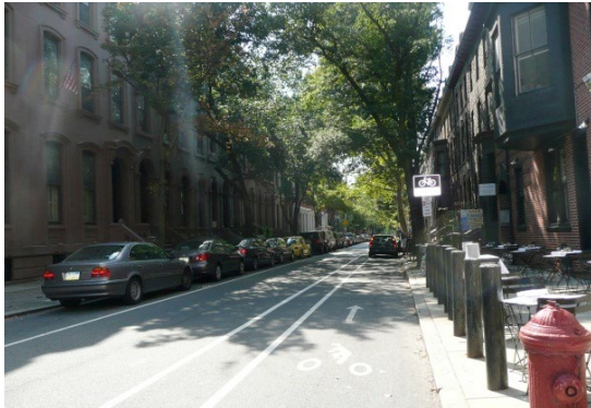
In some areas travel lanes may be removed or narrowed to accommodate complete street facilities.
