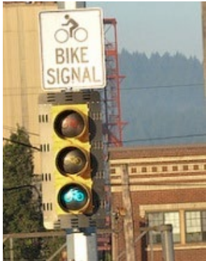
Bicycle signals should be accompanied by a “Bicycle Signal” sign to provide clarification for motorists and cyclists.
