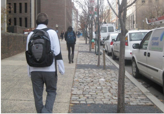
Different pavement treatments can be used to create a pervious walking surface in the furnishing zone. (Note: this space may not count towards ADA clear space requirements.)
