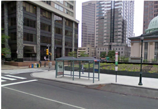
Curb extensions can be used at marked crossings to accommodate stormwater management features, street furniture, bike parking, transit stops, or other features. Above: John F. Kennedy Blvd and 18th St. Below: Queen Lane and McMichael St
