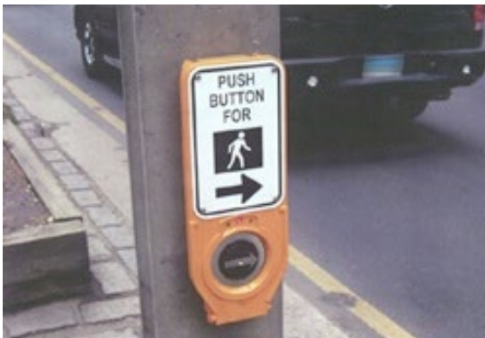
Accessible pedestrian push buttons indicate the WALK sign is lit through sound or other nonvisual signal. Push buttons should be located and signed according to MUTCD and PROWAG standards (MUTCD R10-4) (KAI)
