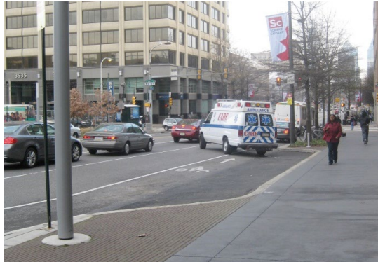
Lay-by lanes should be used rarely because they allow vehicles to encroach into the sidewalk area and decrease comfort and safety for pedestrians.
