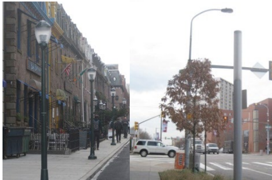
Examples of pedestrian-scale lights and “Brown round” cobra head light (paired with decorative pedestrian – scale light).
