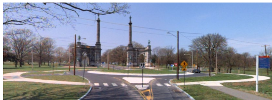
Roundabouts can be used to improve safety and operations at intersections and create new public space, particularly at intersections with complex geometry. (41st Dr and Landsdowne Dr)
