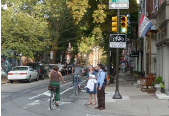
Buffered bike lanes (4.5.3) on Pine Street provide additional protection and comfort for cyclists.
