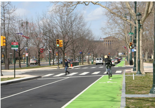
Colored pavement can increase the visibility of bike lanes in areas where parking/stopping in the bike lane is an issue.
