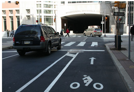
Bike lane word and/or symbol pavement markings should be used to help define buffered bike lanes per MUTCD guidance (MUTCD 9C-3).
