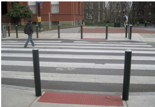
Crosswalks should be at least as wide as the sidewalk, but wider crosswalks can be provided at high traffic areas. (KAI – 34th St south of Walnut St)
