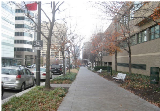
The furnishing zone provides an area for street trees, planters, and green infrastructure.
