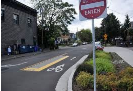
Neighborhood bikeways should incorporate curb extensions, green infrastructure, and other traffic calming features to create a comfortable walking/bicycling environment.
