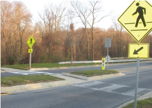
In-street or posted “Yield to Pedestrians” signs (R1-6 or R1-5) and pedestrian warning signs (W11-2) are encouraged at uncontrolled crossings per MUTCD guidance (Source: FHWA)
