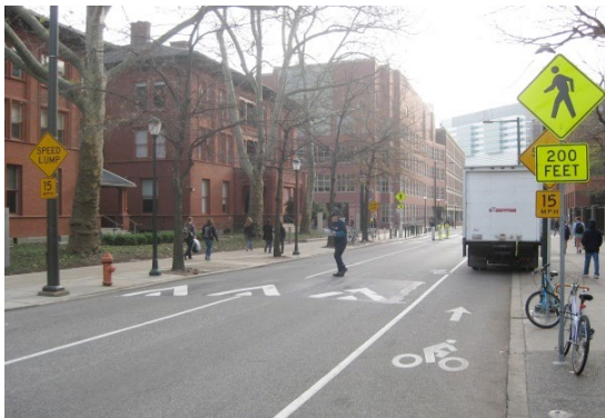
Speed tables are used on 34th Street south of Walnut Street to slow approaching vehicles before a midblock pedestrian crossing.
