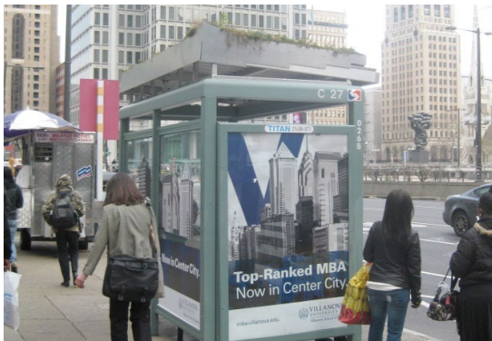
As part of the Green City, Clean Waters plan, the Philadelphia Water Department is piloting a bus shelter green roof at a bus stop near City Hall. (KAI).
