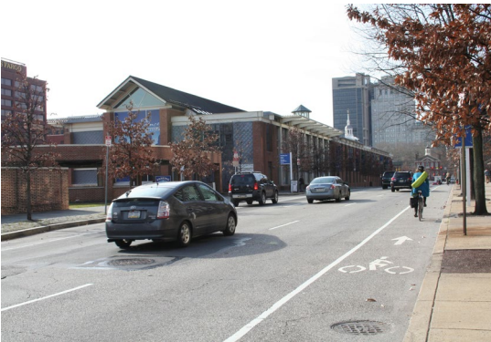
Bike lane word and/or symbol pavement markings should be used to help define bike lanes per MUTCD guidance (MUTCD 9C-3).
