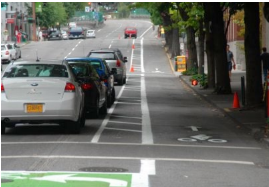
Separated bike lanes may be separated from adjacent travel lanes using parking lanes, raised pavement, planters, or other treatments.
