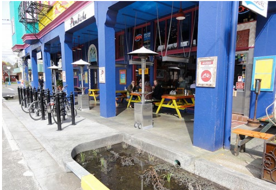
In-street bike parking can be combined with curb extensions to provide a more protected area for bicycles and to accommodate planters or bioswales. (Bikeportland)
