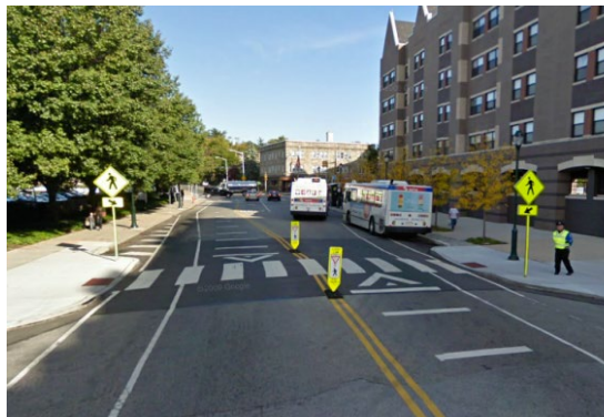
Raised crosswalks should be accompanied by signs and pavement markings to alert motorists of the crossing and pavement change. Detectable warnings should also be used for pedestrians. (54th St south of City Ave)
