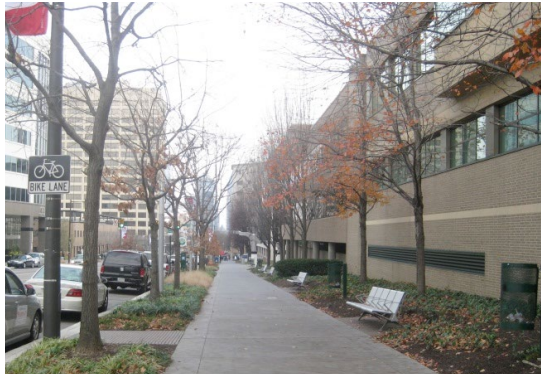
Sidewalk space is typically divided into Building, Walking, and Furnishing zones. The Pedestrian Element primarily addresses the Walking Zone (4.3.2).
