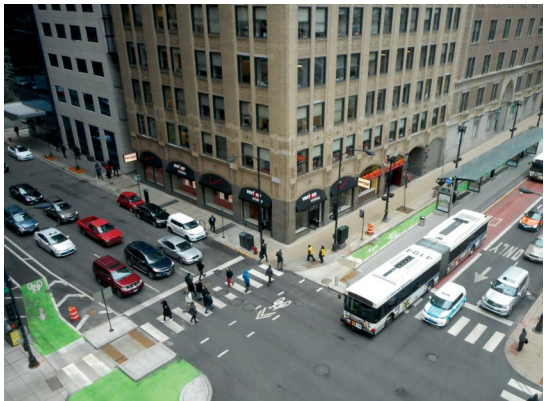
Floating bus stop on Washington Street, Chicago (Source: NACTO)
