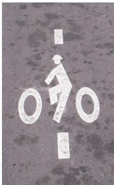
Bicycle detection should be provided at signalized intersections if the phase(s) serving bicycle movements is not set to recall each cycle. The “Bicycle Detector” pavement marking and sign (MUTCD 9C-7 and R10-22) should be used at intersections with in-pavement detectors.
