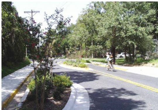
Chicanes are used for traffic calming and stormwater management, particularly near parks in Portland, OR. (streetsblog).
