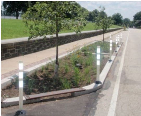
Stormwater bump-outs provide the pedestrian crossing benefits of curb extensions and help manage stormwater overflow.
