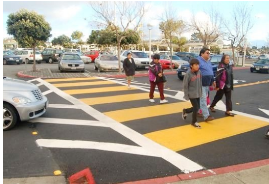
Raised crosswalks provide a level, highly visible crossing for pedestrians and traffic calming for vehicles. (Streetsblog SF)
