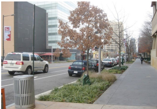
Tree trenches can accommodate multiple trees and may be connected to an underground infiltration structure.
