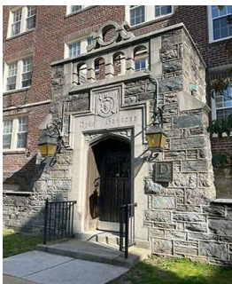
Central wing entrance showing original sconces: Libbie Hawes
