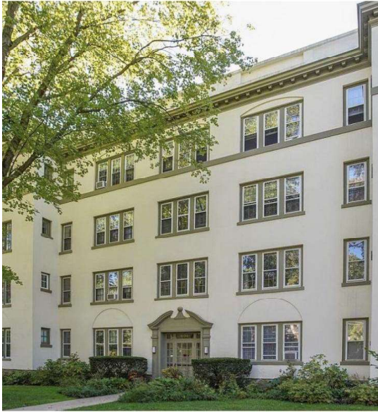
Entry Facade: Adrienne Carpenter
