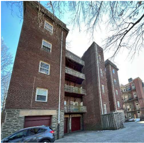
Rear Stair Towers: Libbie Hawes
