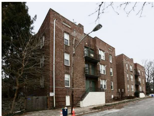
South Corner View: apartments.com
