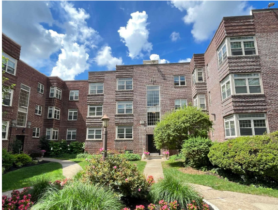
Entrance to Building A from courtyard
