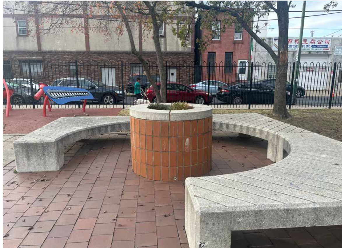
Existing benches and planters to be removed
