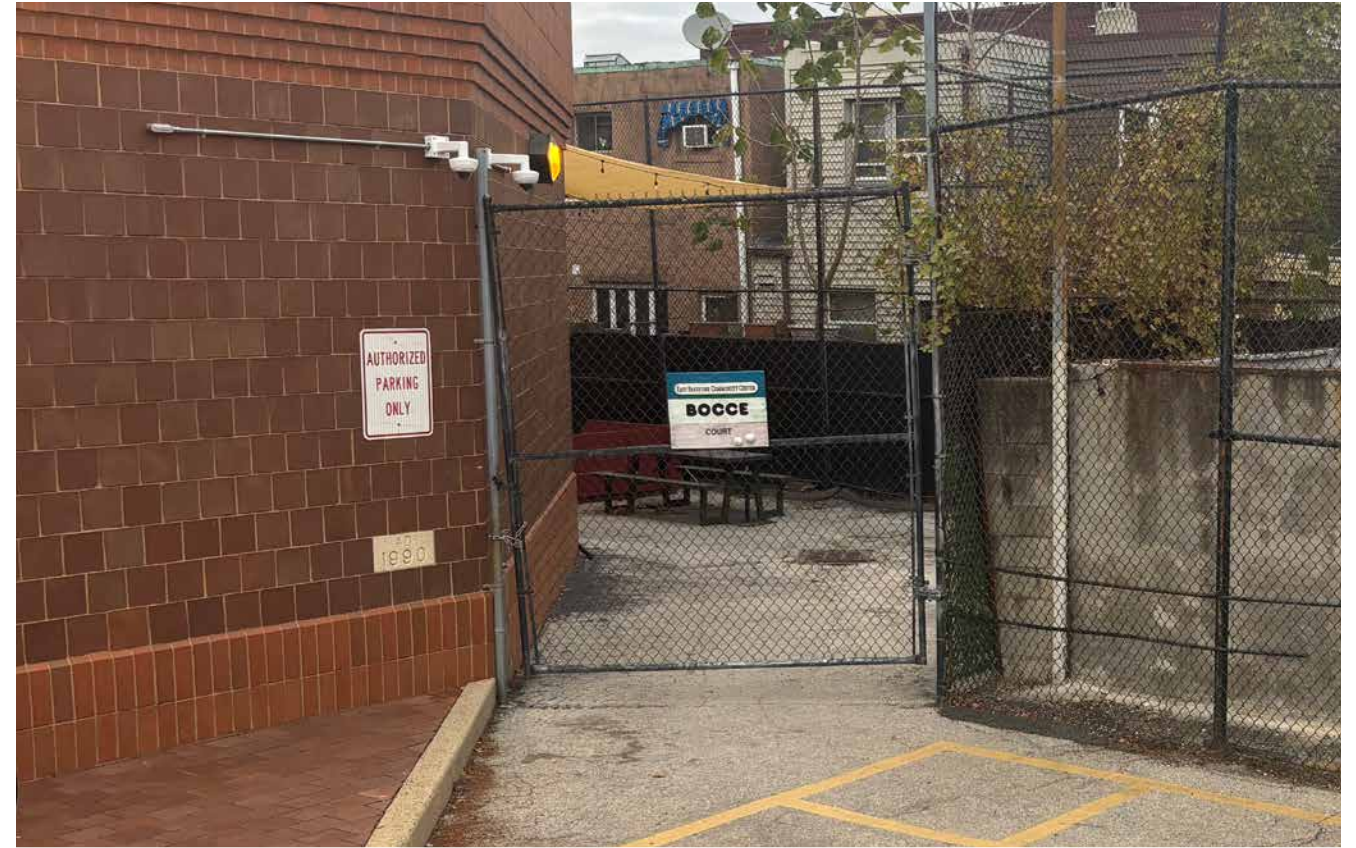
Existing gate to bocce area to be replaced
