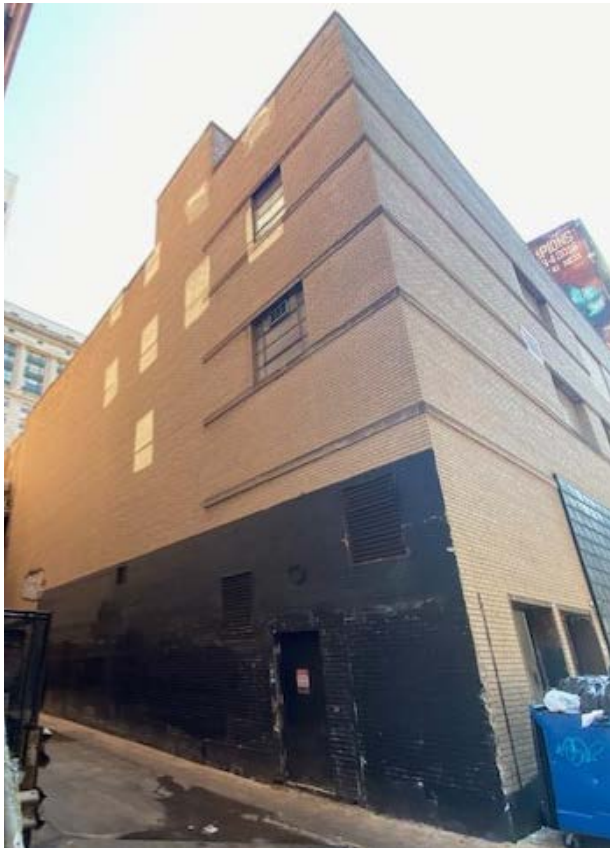
Figure 4. West facade of 1330-36 Chestnut Street, August 2023.
