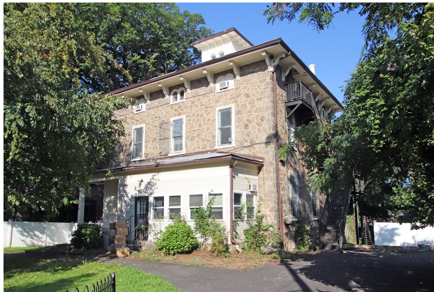
Figure 1: South and east elevations, looking northwest from Locust Avenue. Photo taken August 13, 2024.
