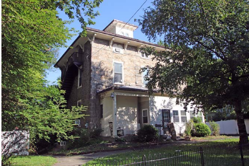
Figure 2: South and west elevations, looking northeast from Locust Avenue. Photo taken August 13, 2024.
