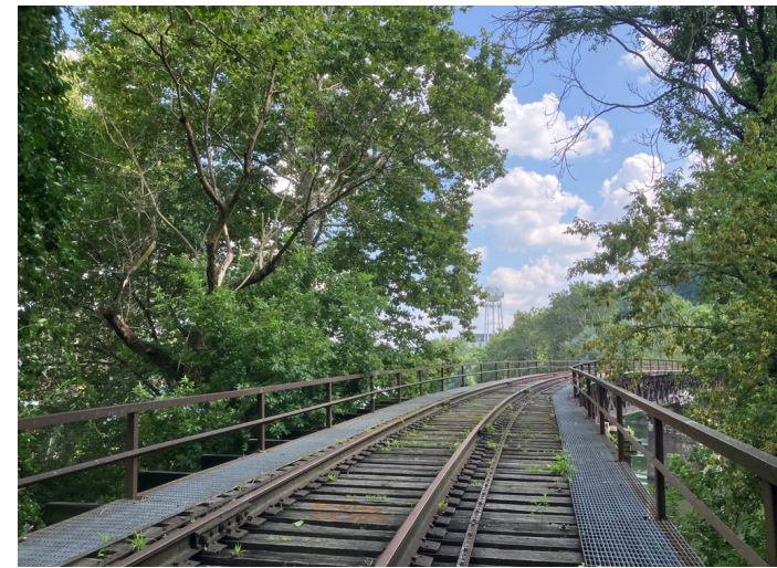
Existing Mule Bridge, currently in planning phase | City of Philadelphia
