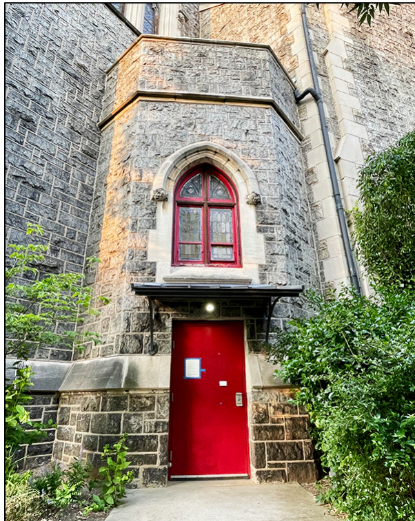
Fig. 11. Entry door for office along S. 48 th Street.
