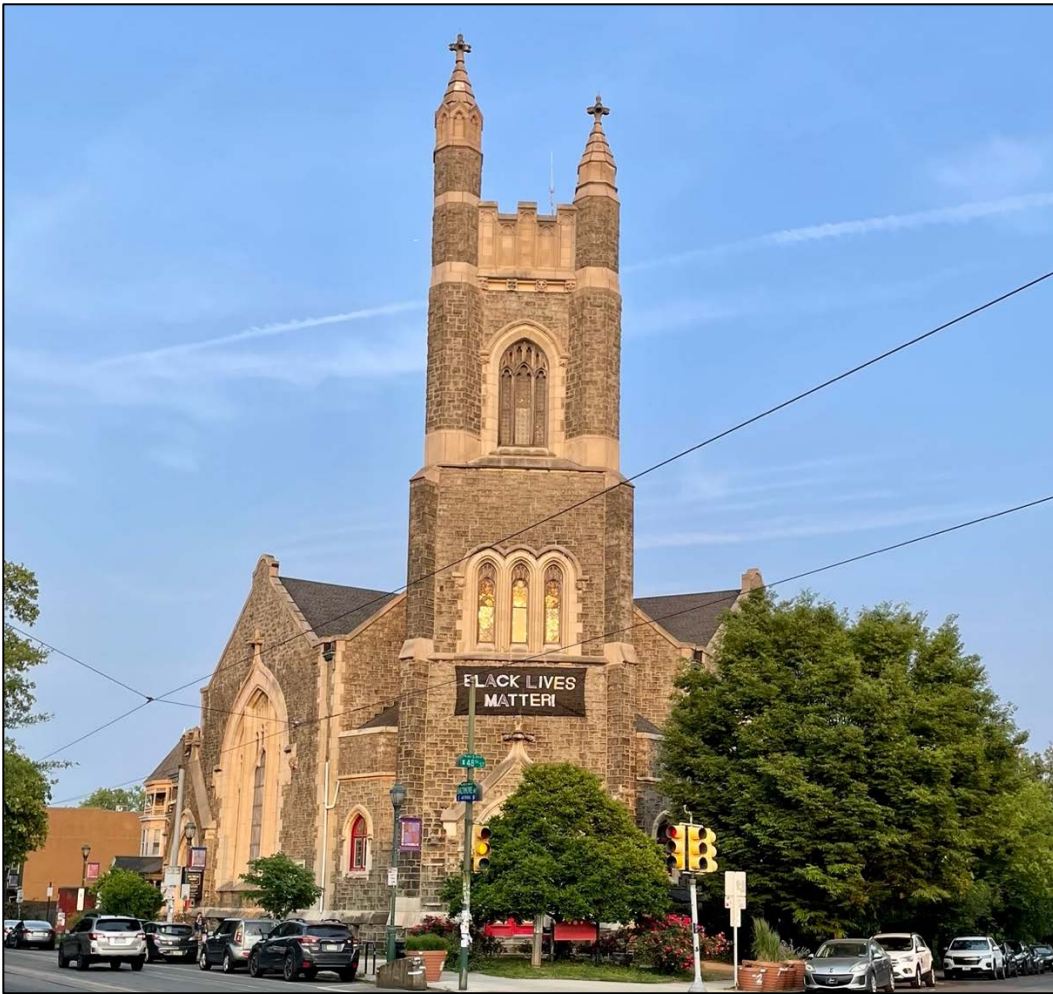
Fig. 4. Primary elevation of at S. 48 th Street & Baltimore Avenue.
