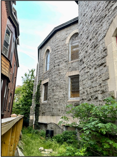
Fig. 12. Rear of building at Baltimore Avenue.
