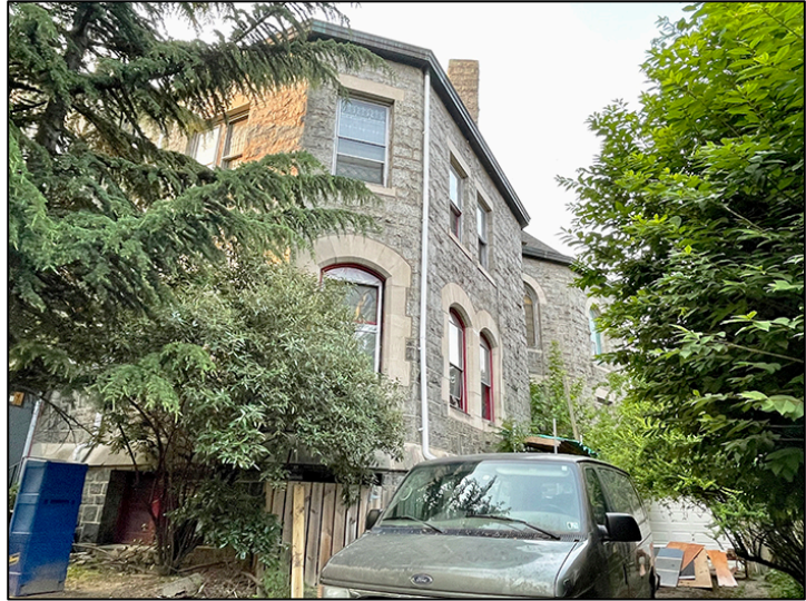
Fig. 13. Rear of building at S. 48 th Street at the west elevation.
