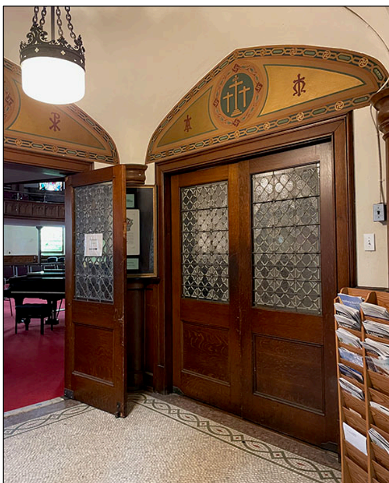
Fig. 27. Interior doors with decorative leaded glass lights, mosaic floors, original light fixture and painted transom details. Note that no interior designation is included as part of this nomination.
