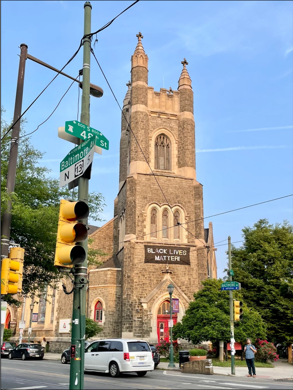
Fig. 5. Primary (northwest) elevation dominated by the granite tower and taller corner spirelet within the wedge of the five-point street intersection.
