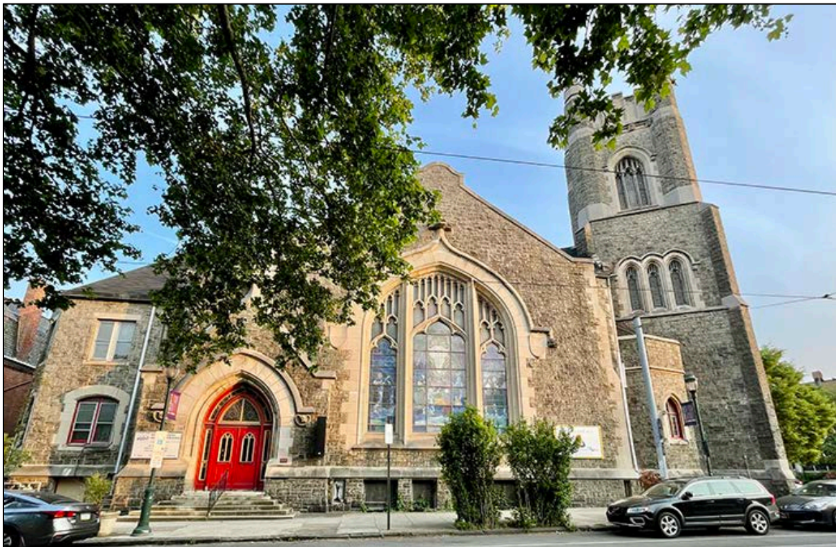
Fig. 6. North elevation along Baltimore Avenue.
