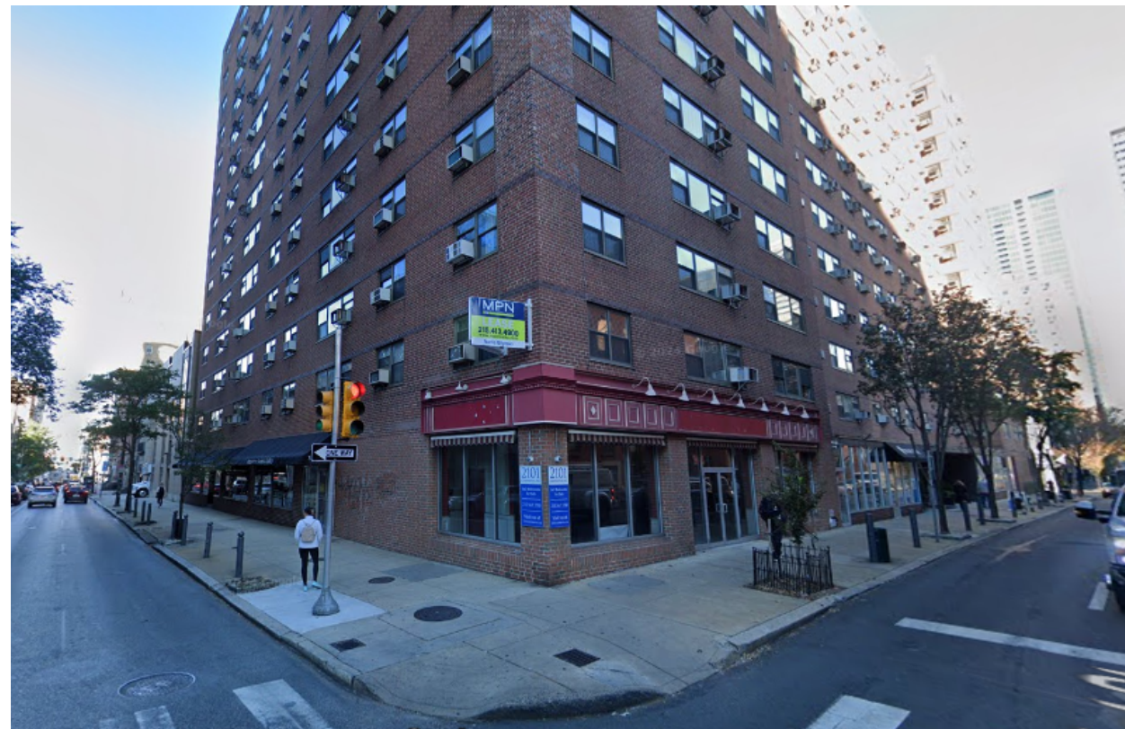
2101 Walnut St. looking North on 21st St
