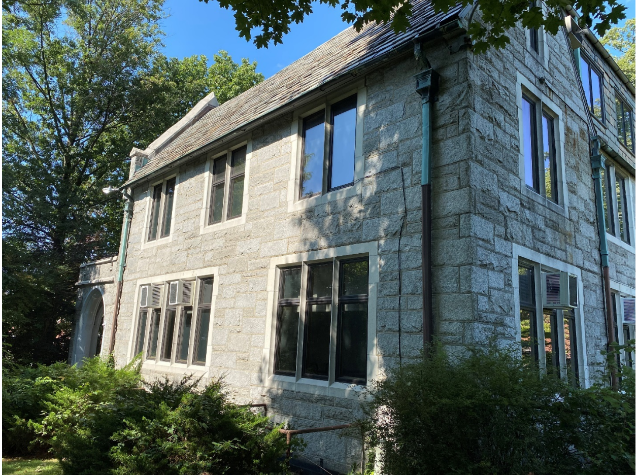
Figure 10. East façade. Source: Nominator.
