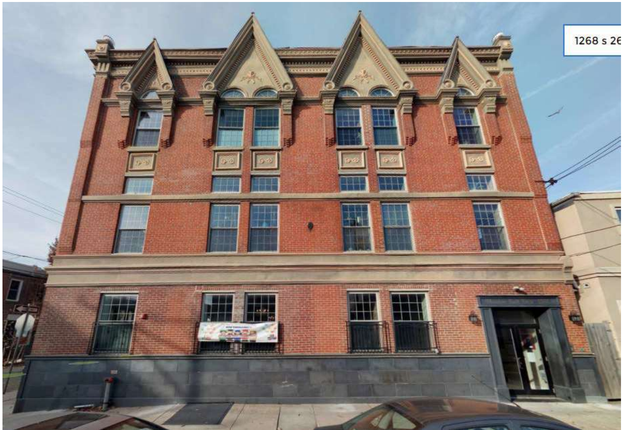
Figure 3: East façade of 1268 S 26 th Street facing West. Source: Cyclomedia.phila.gov
