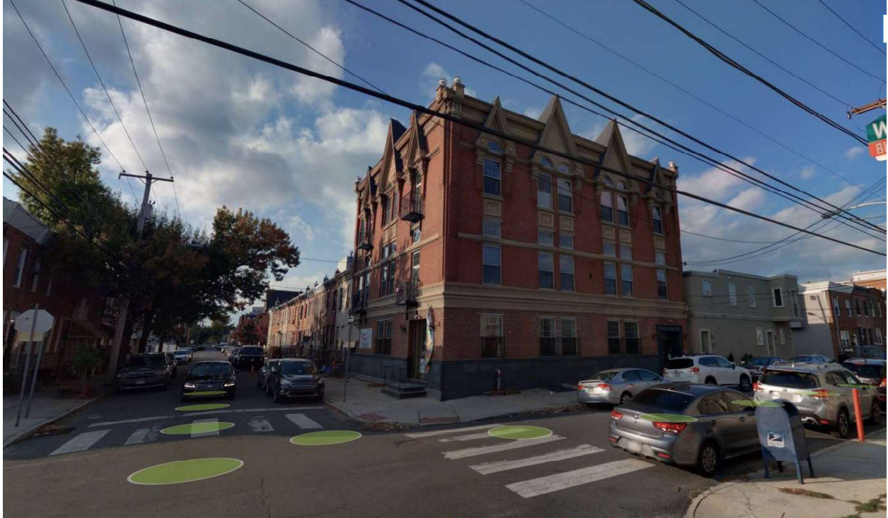
Figure 7: Wharton Hall shown in context with the surrounding rowhouses. Source: Cyclomedia.phila.gov
