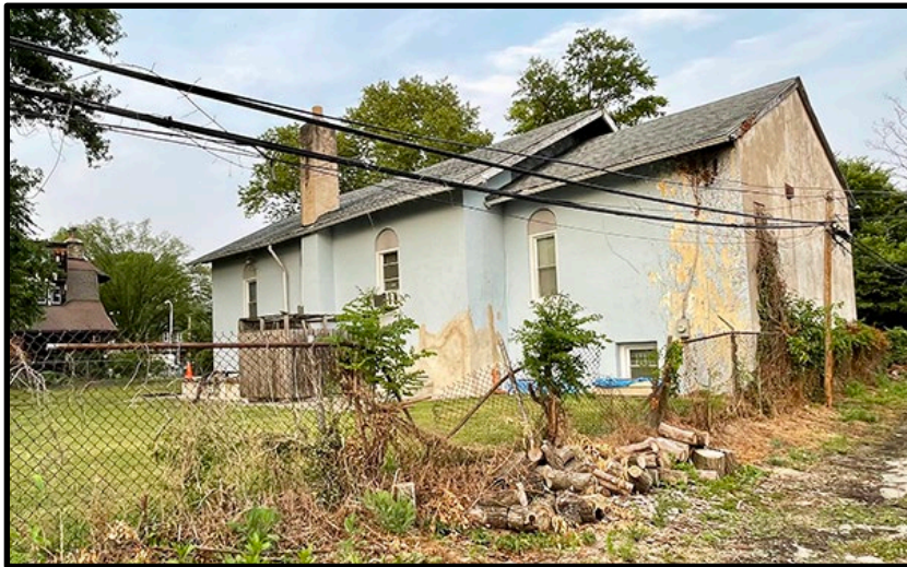
Figure 5. The rear, alleyway elevation of the barn.
