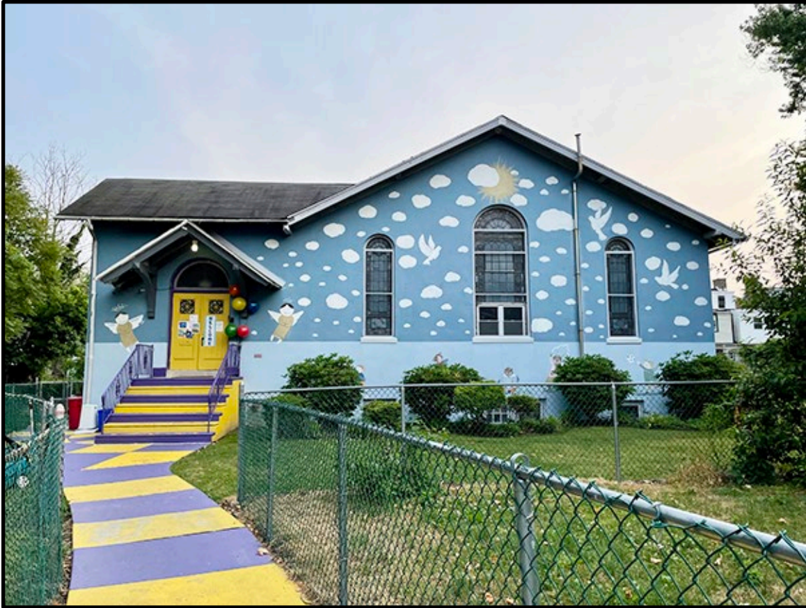
Figure 2. The northeast and primary elevation of the Sallie Watson Barn that later became the church and parish hall for the First Presbyterian Church of Germantown.
