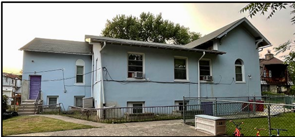
Figure 4. The southeast elevation of the barn and former church.
