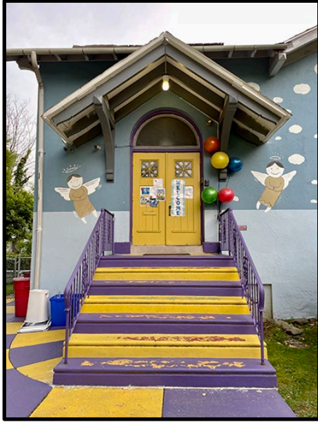
Figure 3. The main entry point into the former Presbyterian church.
