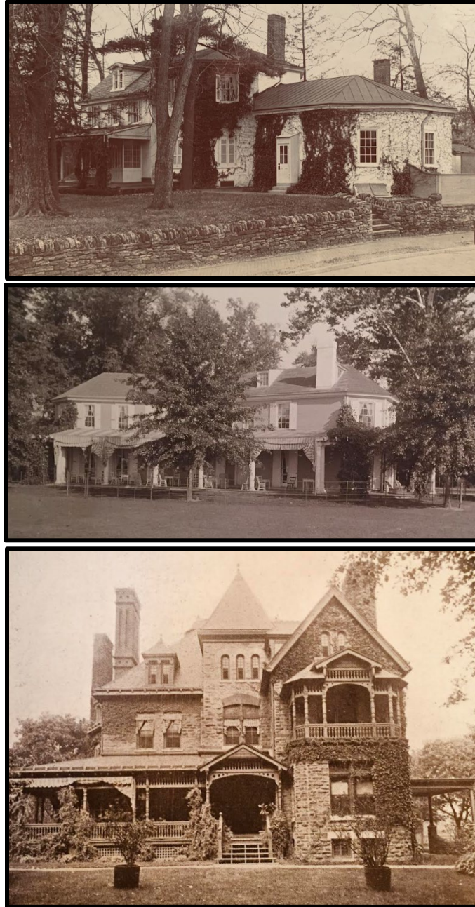
Figure 12. Top: "White Cottage" was an eighteenth-century house with early nineteenth century additions on the northerly side of Manheim Street between Greene Street and Wayne Avenue that was demolished in ca.1907 for 88 row houses. Source: Germantown Historical Society. Figure 13. Middle: "Caernarvon," the Wister Price House, Manheim Street, Germantown, later the Ladies Club House of the Manheim Cricket Club, now the Germantown Cricket Club. Source: Shoemaker Collection, Historical Society of Pennsylvania. Figure 14. Bottom: The Residence of Samuel A. Hendrickson, at the northeast corner of Manheim and Morris Streets. Source: Germantown Historical Society.
