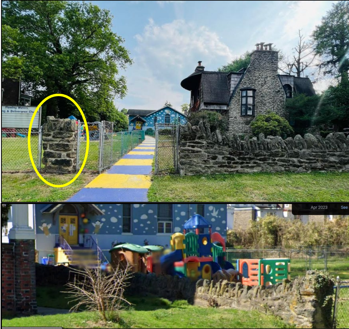
Top: Figure 7. Schist Boundary Wall from Wayne Avenue.
