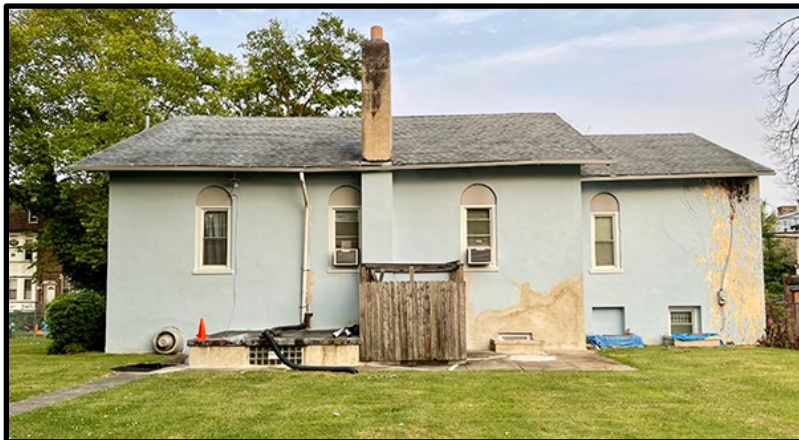
Figure 6. The northwest elevation of the barn.
