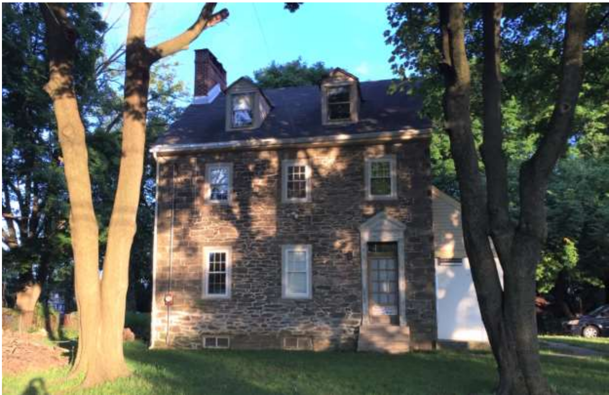
Figure 2: Front elevation, July 2022, David Nepley. Note the original plank frames supporting the window openings. Replacement windows replicate what is likely the original six-over-six divided-lite configuration.
