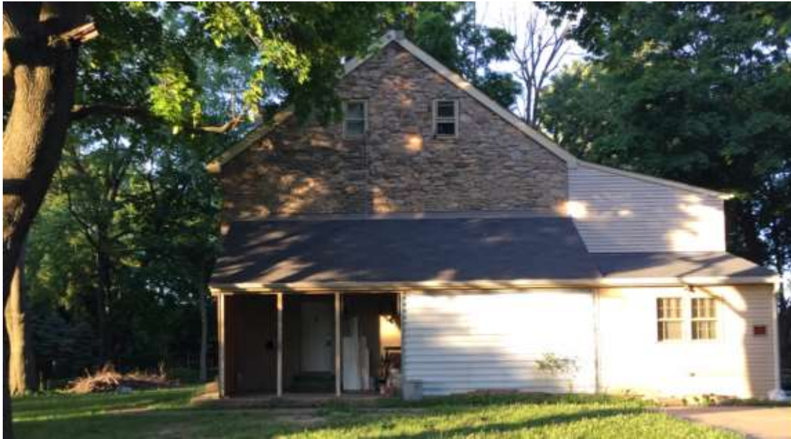
Figure 5: Southwest side elevation, July 2022, David Nepley.
