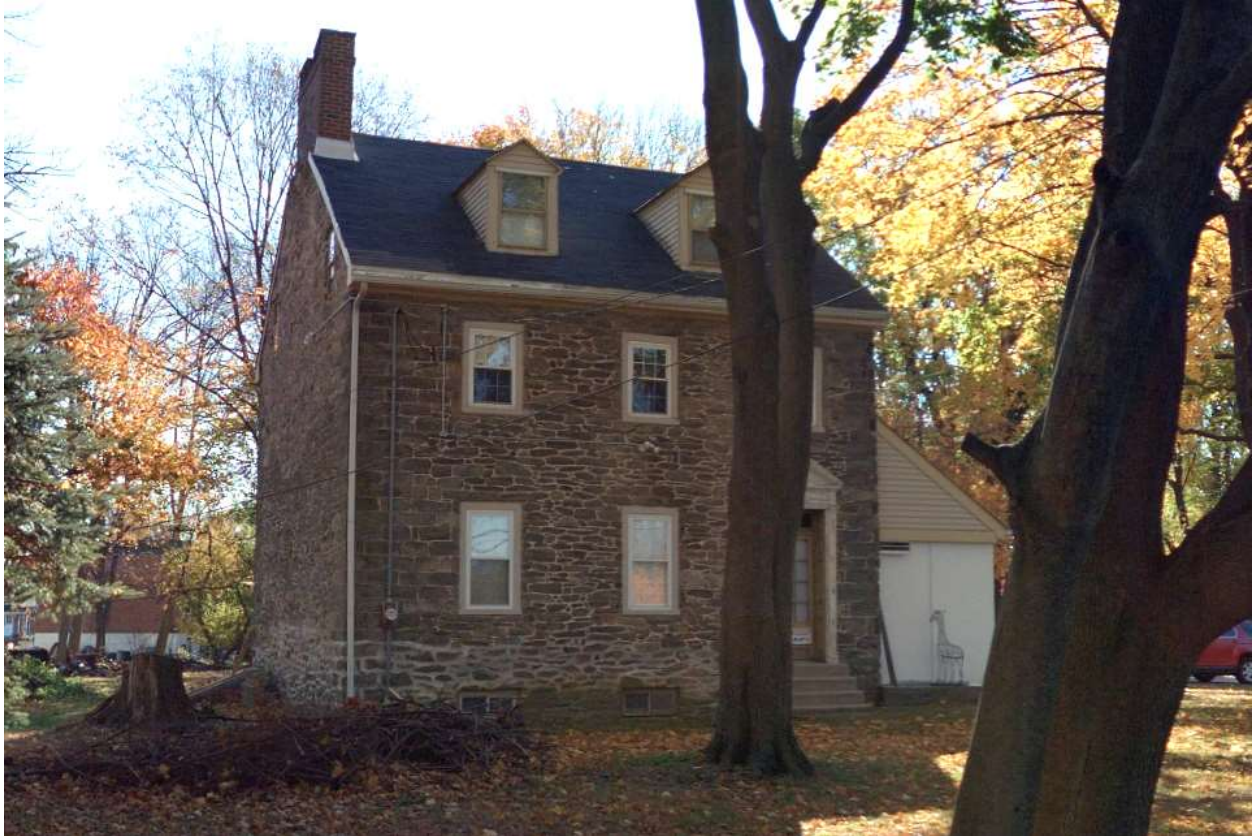
Figure 8: Front and northeast side elevation. Source: David Nepley, July 2022.
