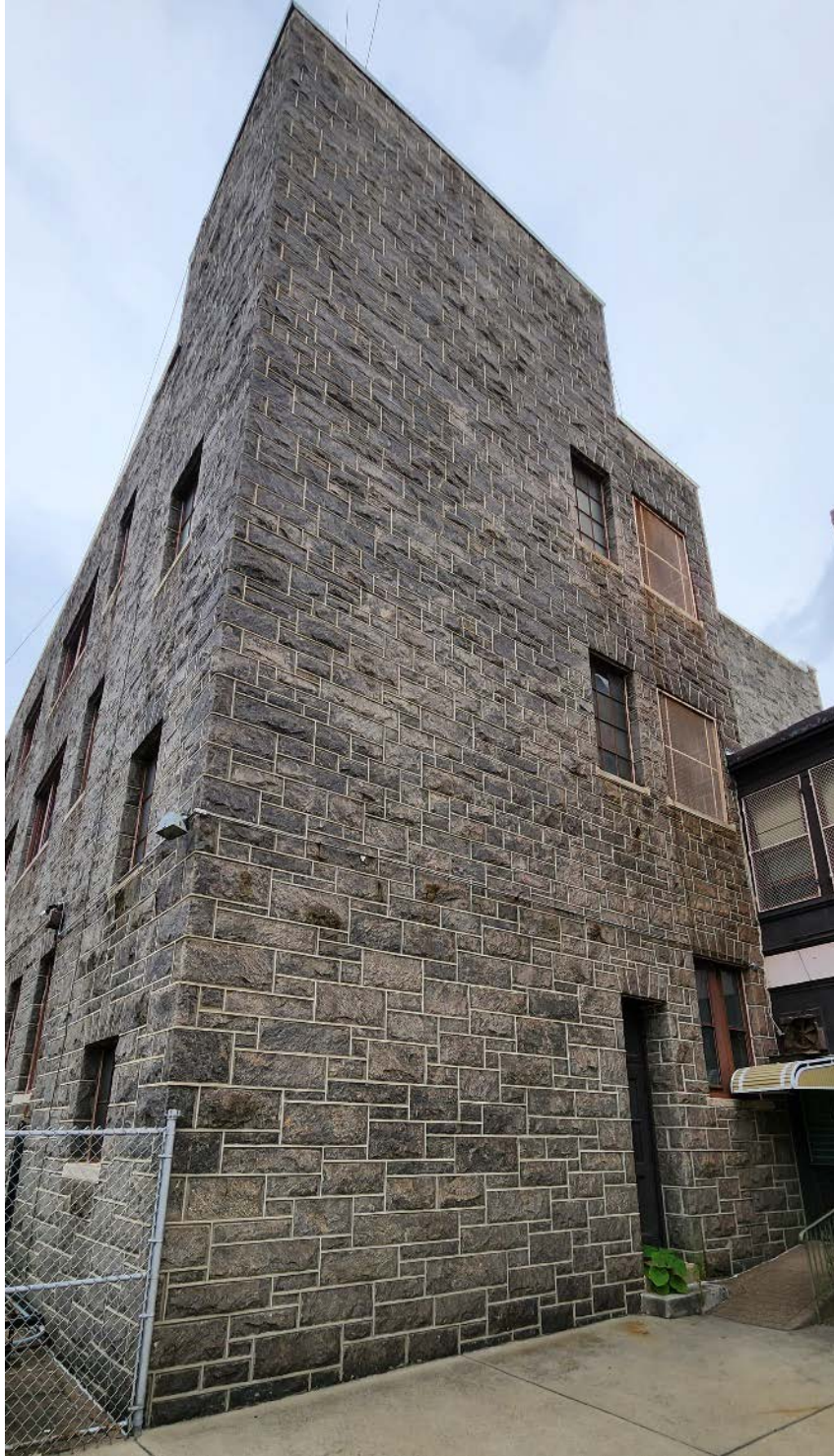
Figure 5: North Elevation facing courtyard. Photo: Dennis Carlisle
