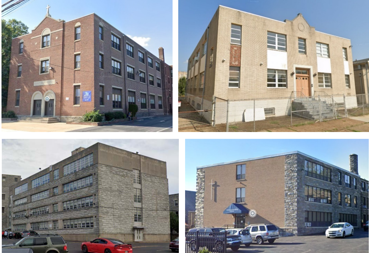
Figure 9: Left to Right, 1 st Row: Saint Bernadette School, 1001 Turner Road, Drexel Hill, PA, 1948. Immaculate Conception School, 811 N 8 th Street, Philadelphia, PA, 1951. 2 nd Row: Saint Martin School Annex, 5400 E Roosevelt Boulevard, Philadelphia, PA, 1956. Annunciation B.V.M. School Addition, 421 Brookline Boulevard, Havertown, PA, 1958. Photos: Google Streetview.
