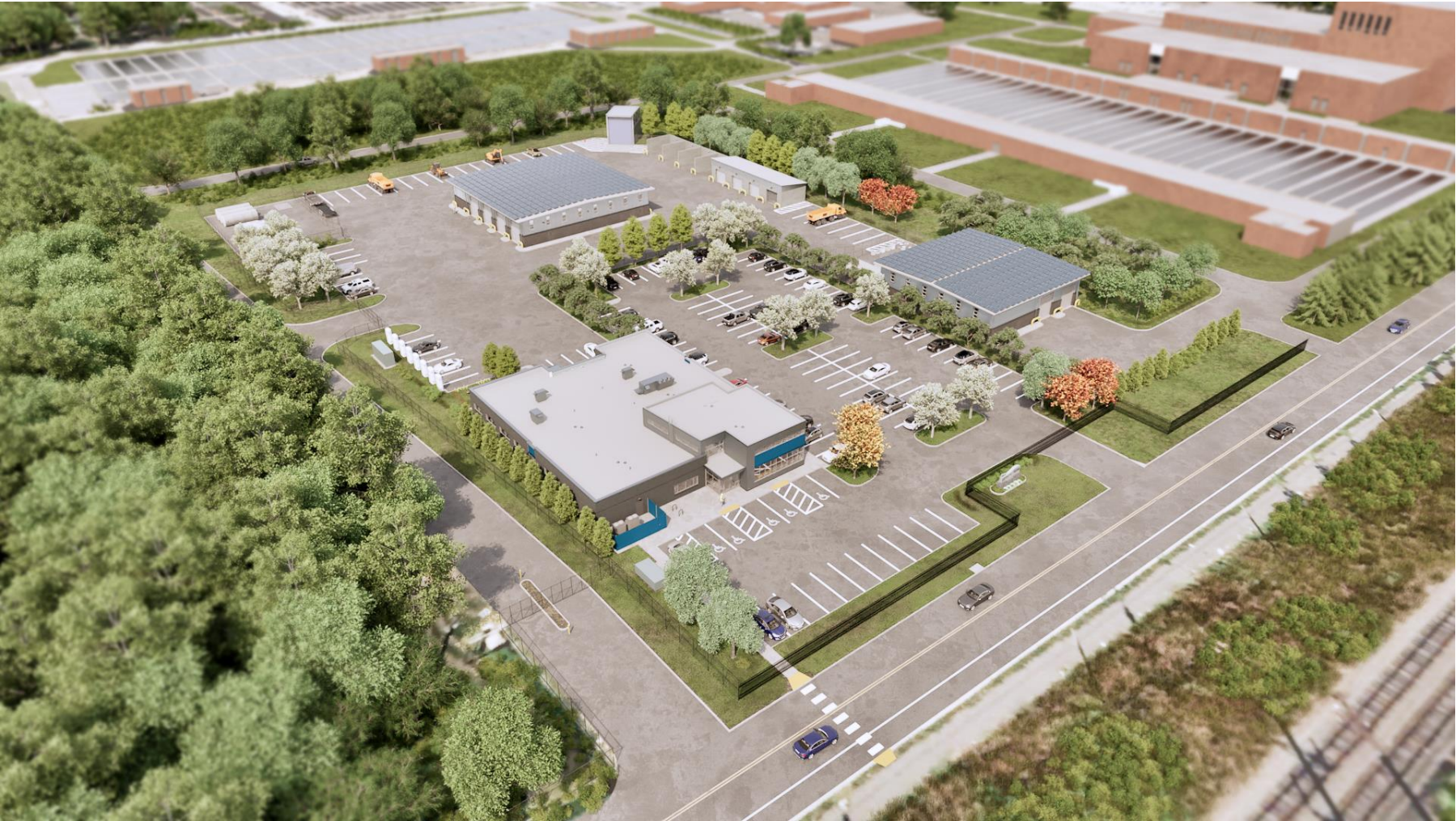
Aerial View from Southeast Corner of Site
