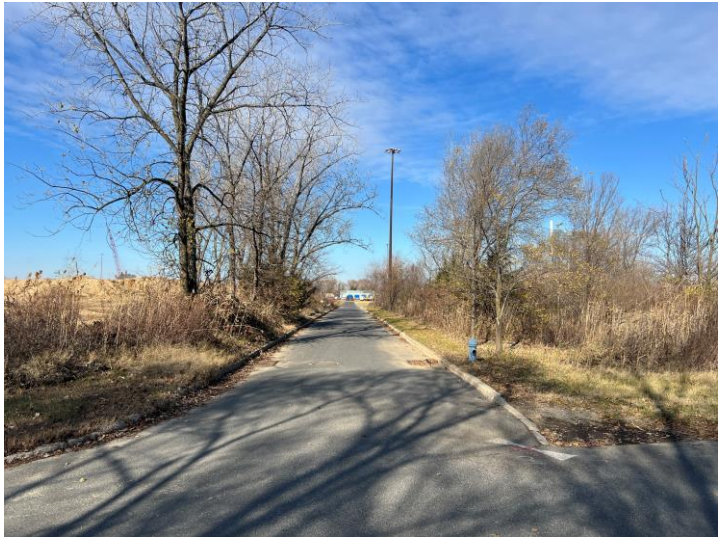
View Looking North From Road C/Road H
