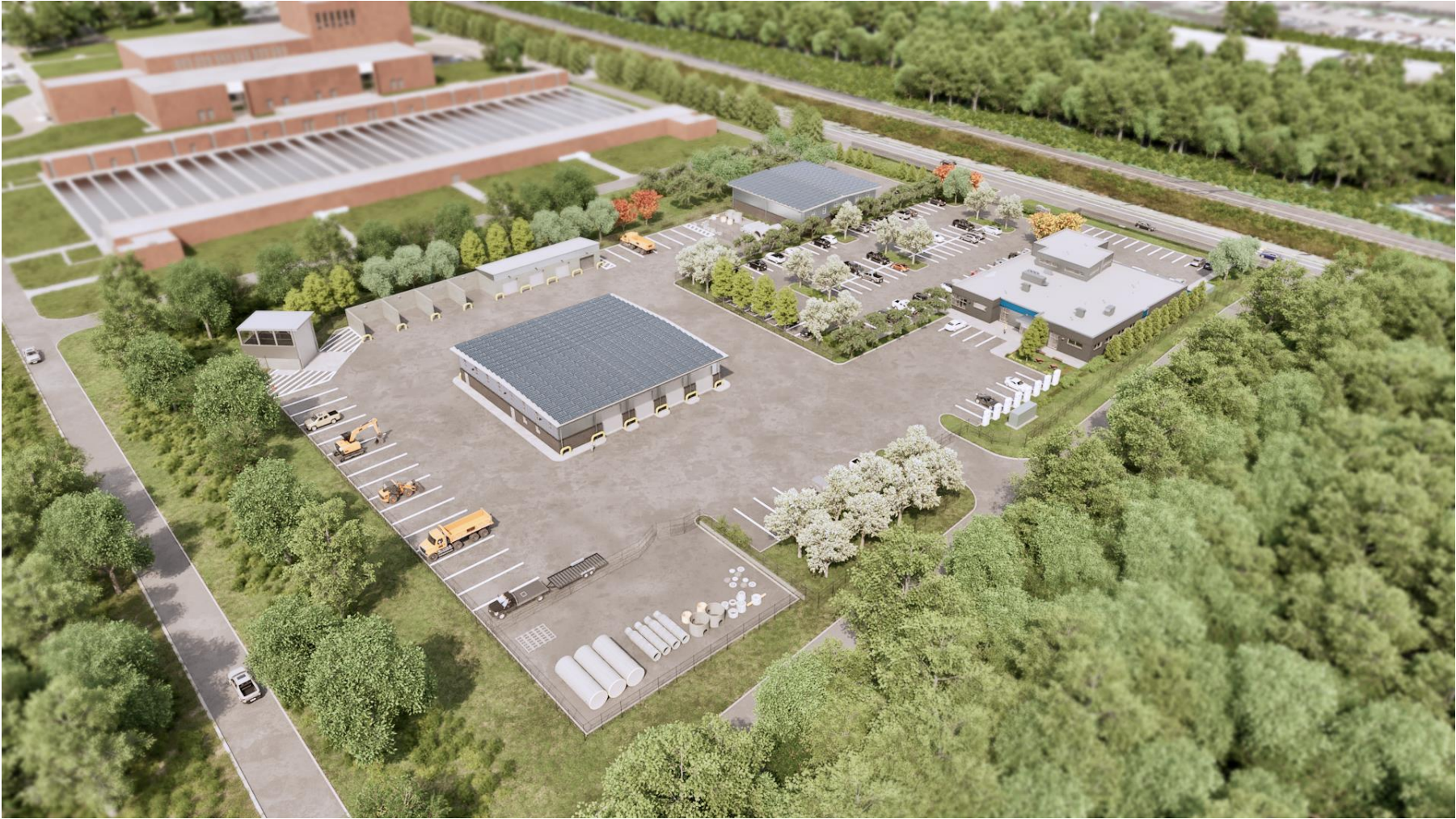
Aerial View from Southwest Corner of Site
