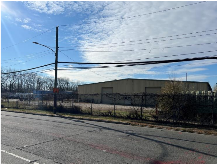
View Looking West On Lewis Street Near Road G Site Entrance
