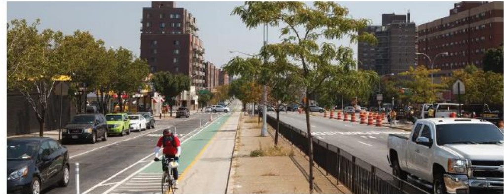
Queens Boulevard, New York City, with inner & outer lanes
