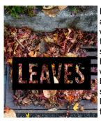
Leaves can cause a clogged inlet, which could cause flooding on the street during heavy rains. PWD will clean the inlet, but neighbors should ensure that leaves and other trash is cleared.
