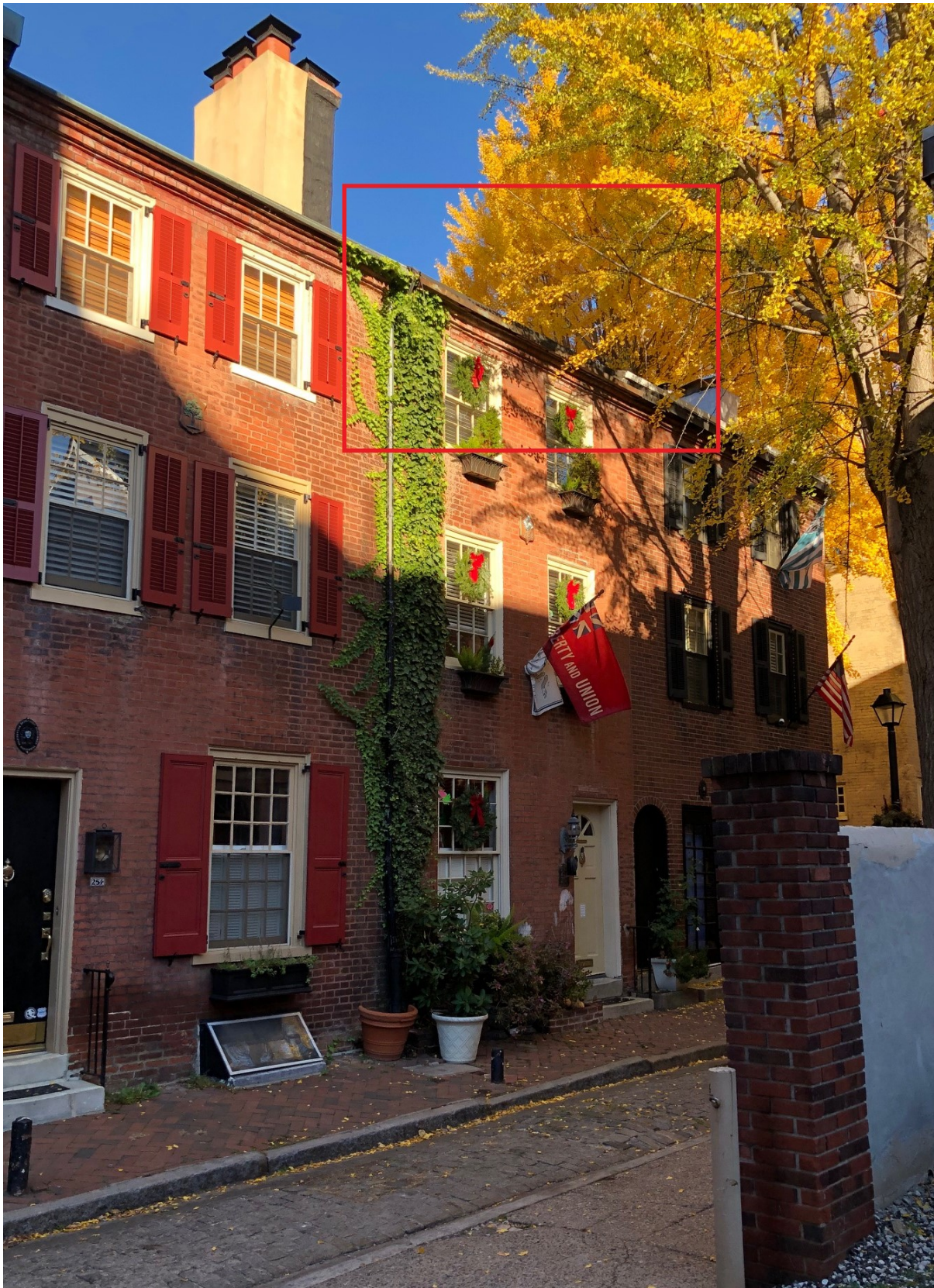
Figure 6: Front façade of 252 Quince Street, December 2023.
