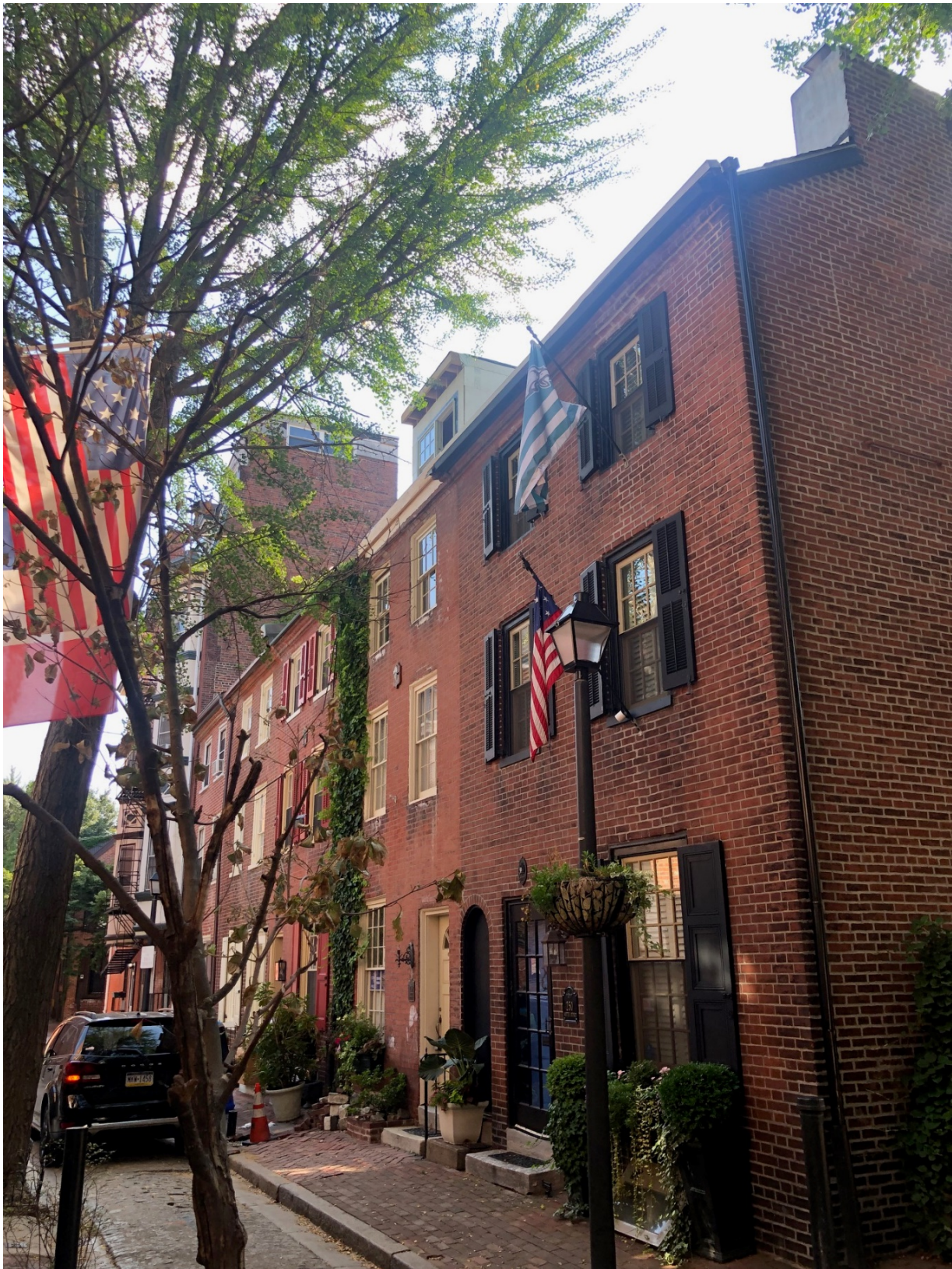
Figure 4: 200 Block of Quince Street in August 2024 while under construction. 250- 258 252 Quince Street is second from right in the image.
