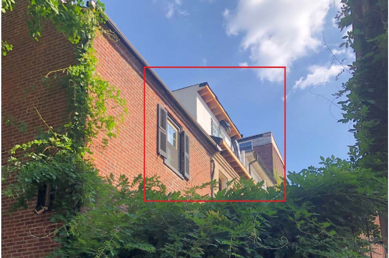
Figure 9: Rear façade of 252 Quince Street as viewed from Manning Street, August 2024.
