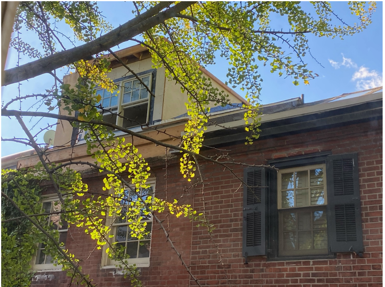
Figure 2: As built condition of front roof, November 2024.
