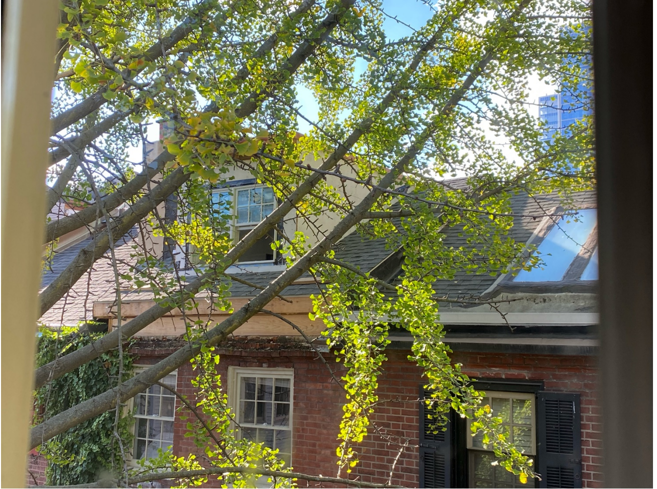
Figure 1: As built condition of front roof, November 2024.
