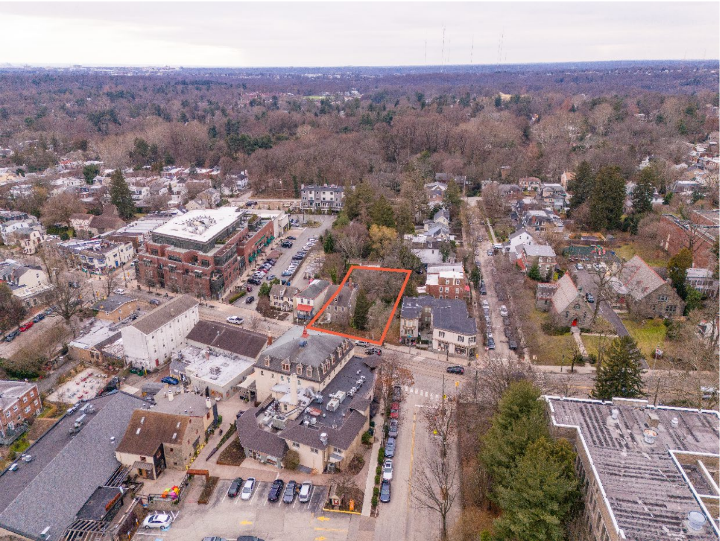
EXISTING AERIAL 2 : EAST
