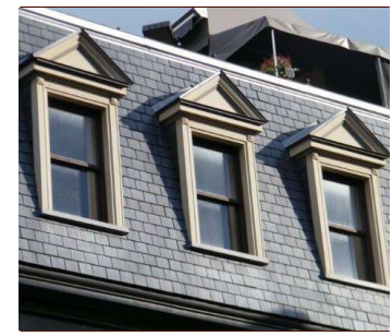
2. SLATE SHINGLE ROOF
