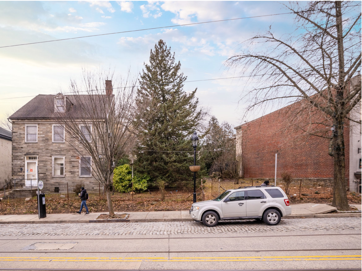
SITE PHOTO 2: LOOKING AT EAST SIDE OF THE SITE
