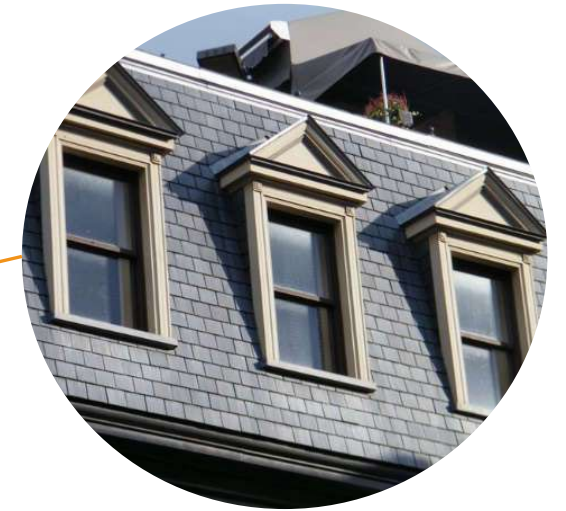
SLATE SHINGLE ROOF
