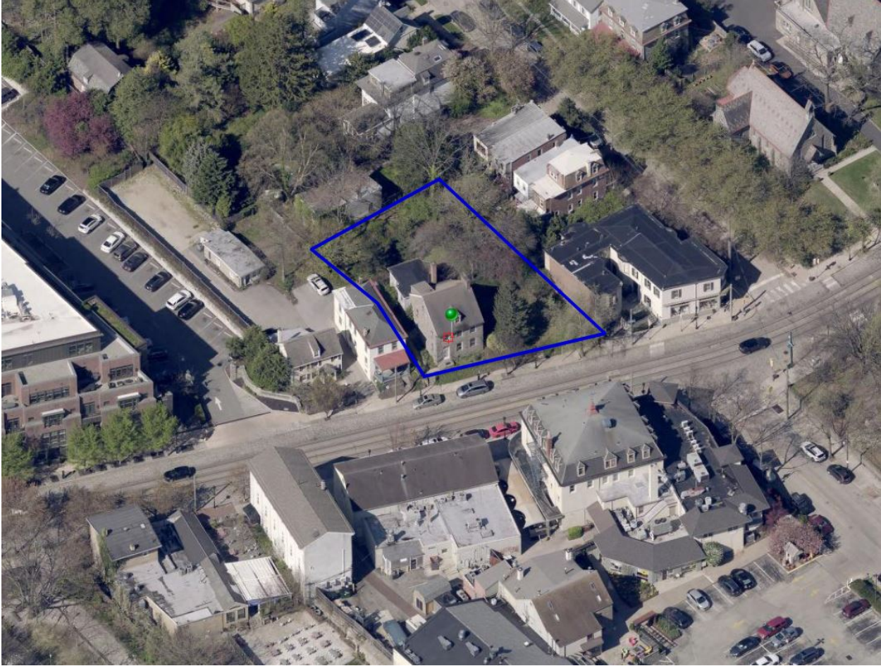
Figure 3: Aerial view of 8226 Germantown Ave, looking west:
