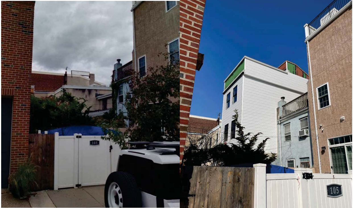
Left: Photo of 1108 S Front Street on 10/9/2023 (Cyclomedia); Right: Photo taken 3/14/2024 by PHC staff.
