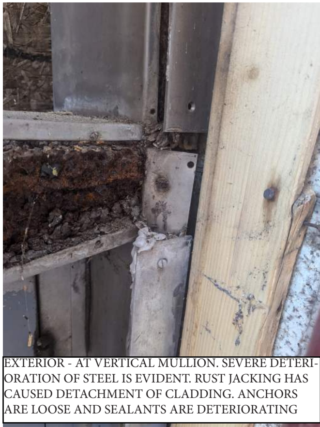
EXTERIOR - AT EAST VERTICAL MULLION. RUST JACKING HAS CAUSED DETACHMENT OF CLADDING. ANCHORS ARE LOOSE AND SEALANTS ARE DETERIORATING.
