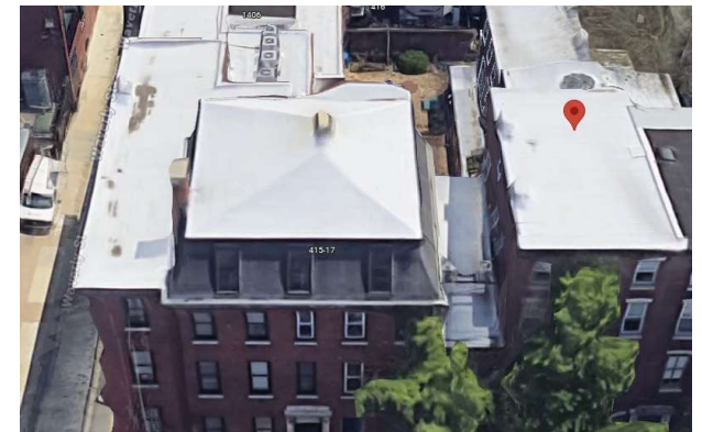
D Aerial view illustrating existing masonry openings and non-original dormer windows along the north side of 419 S 15 th Street, along with the non-original asphalt shingles on the mansard roof. Original cornice line to be maintained with an 15'-9" setback along 15 th Street.
