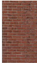
Restored Original Brick w/ limited matching infill
