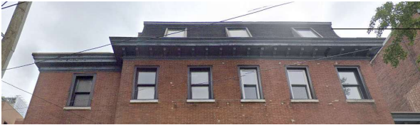
Paint and Restore original cornice; repair mansard roof as required
