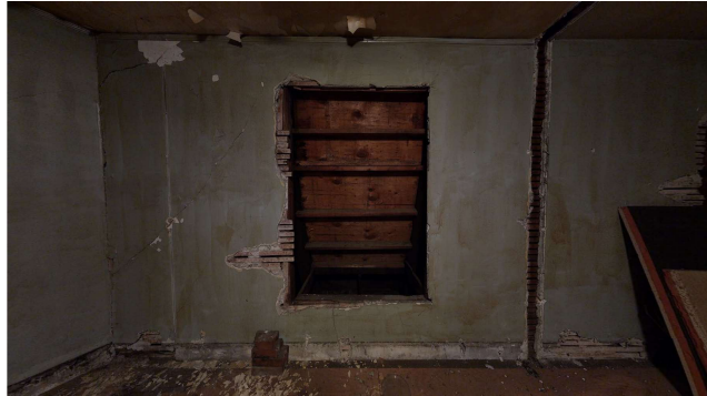
A Opening in existing mansard roof, illustrating non-original plywood roofing sheathing; It is assumed that entire roof has been replaced including asphalt shingles and plywood sheathing. Original framing members are still present; removal will be minimized to the opening itself.
