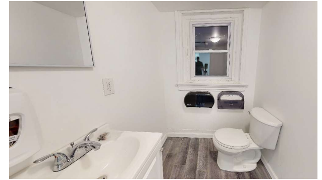
B Existing 4 th floor masonry opening at location of connector, present in 419 S 15 th Street; visible from interior and exterior.
