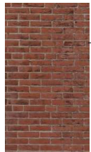
Restored Original Brick w/ limited matching infill
