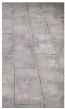
Concrete Landscape Pavers in Courtyard
