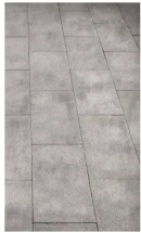
Concrete Landscape Pavers in Courtyard
