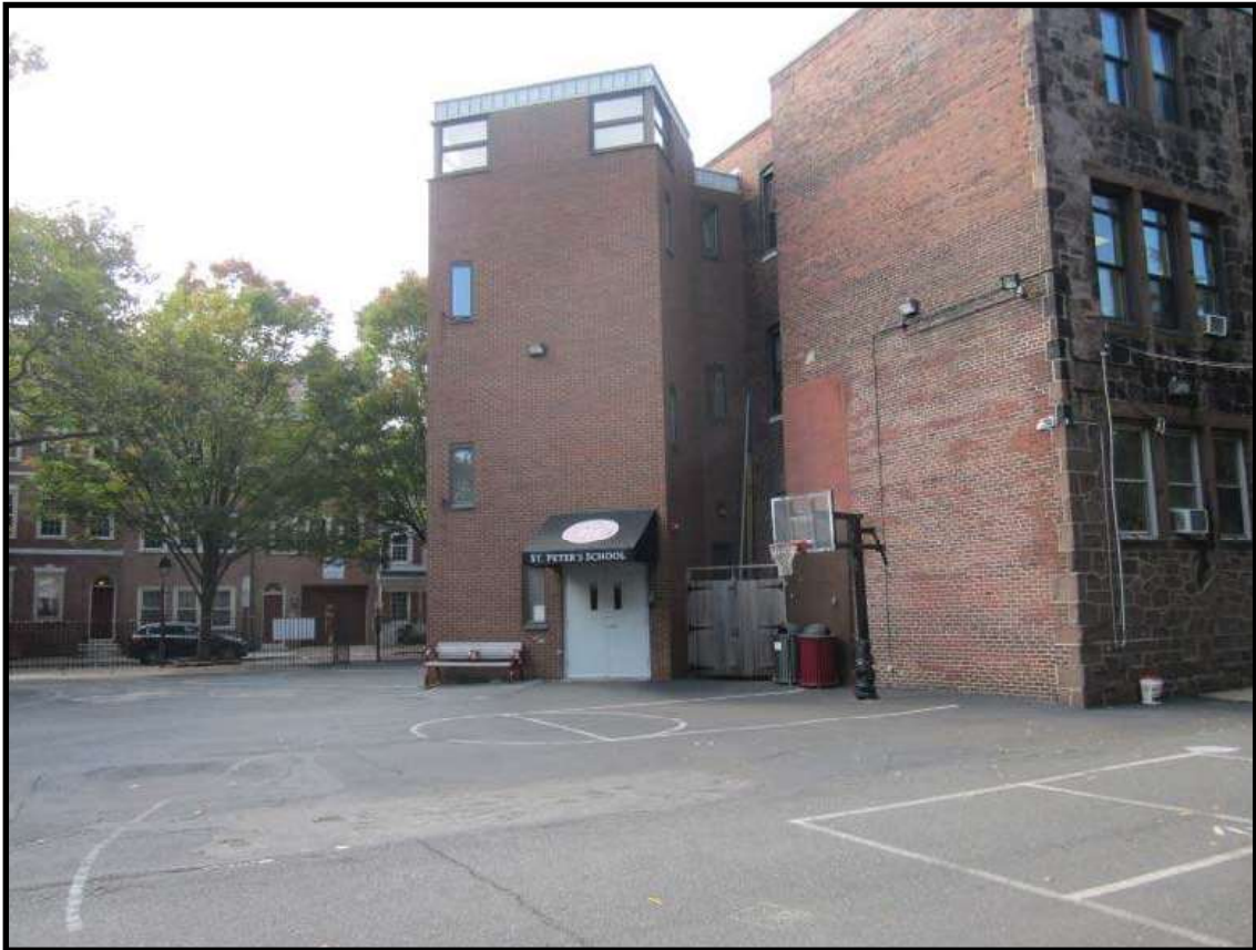
Photograph 3.5. Proposed site of St. Peter's Parish Hall, corner of Third and Lombard Streets, view of western end of site looking south from northern edge of Parcel B; St. Peter's School at right (Photographer: Richard Hunter, October 2016) [HRI Neg. #16054/D1:019].
