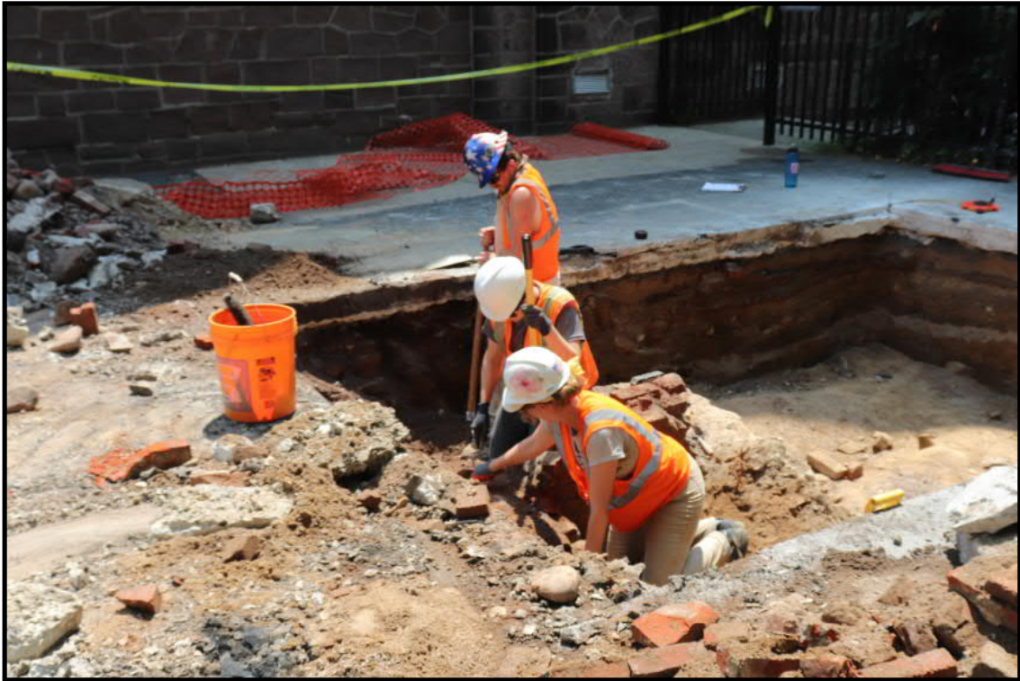
Photograph 3.2. View facing southwest showing manual clearing of the pricy feature in Test Pit A (Photographer: Andrew Martin, July 2019) [HRI Neg.# 19027/D1:111].
