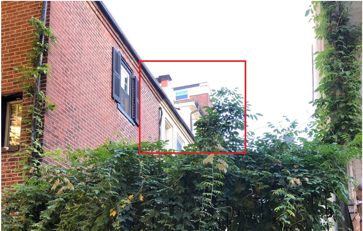
Figure 8: Rear façade of 252 Quince Street as viewed from Manning Street, December 2023.
