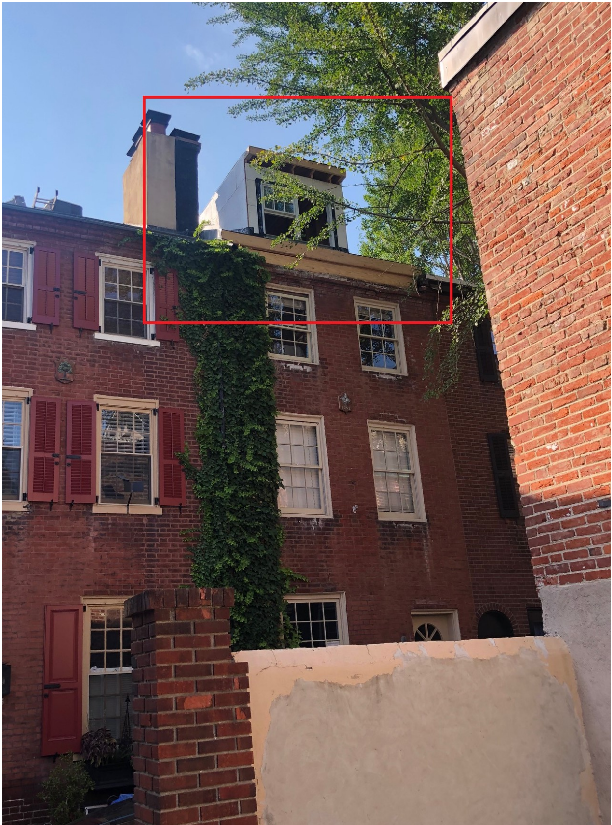
Figure 7: Front façade of 252 Quince Street, August 2024.
