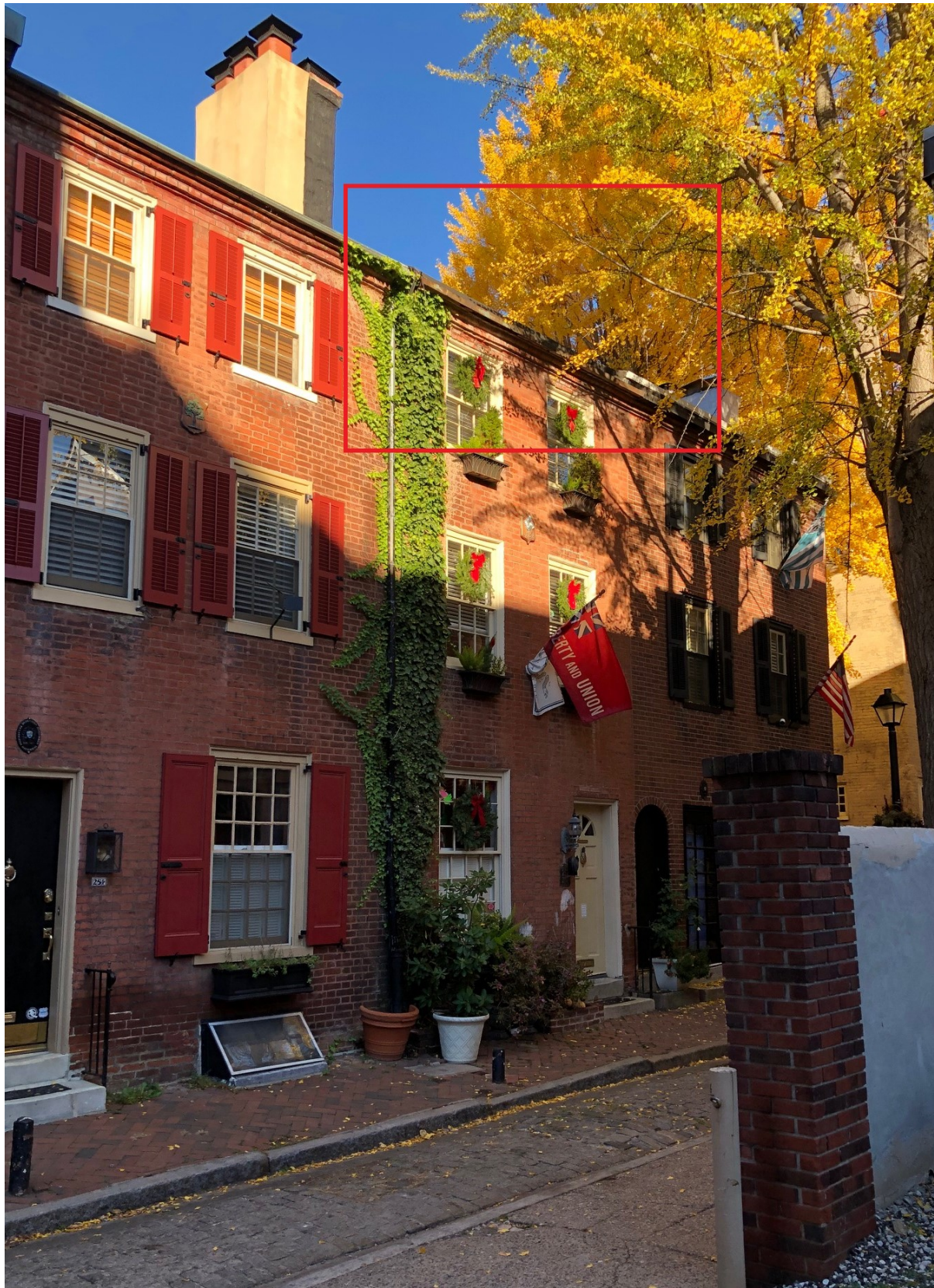
Figure 6: Front façade of 252 Quince Street, December 2023.
