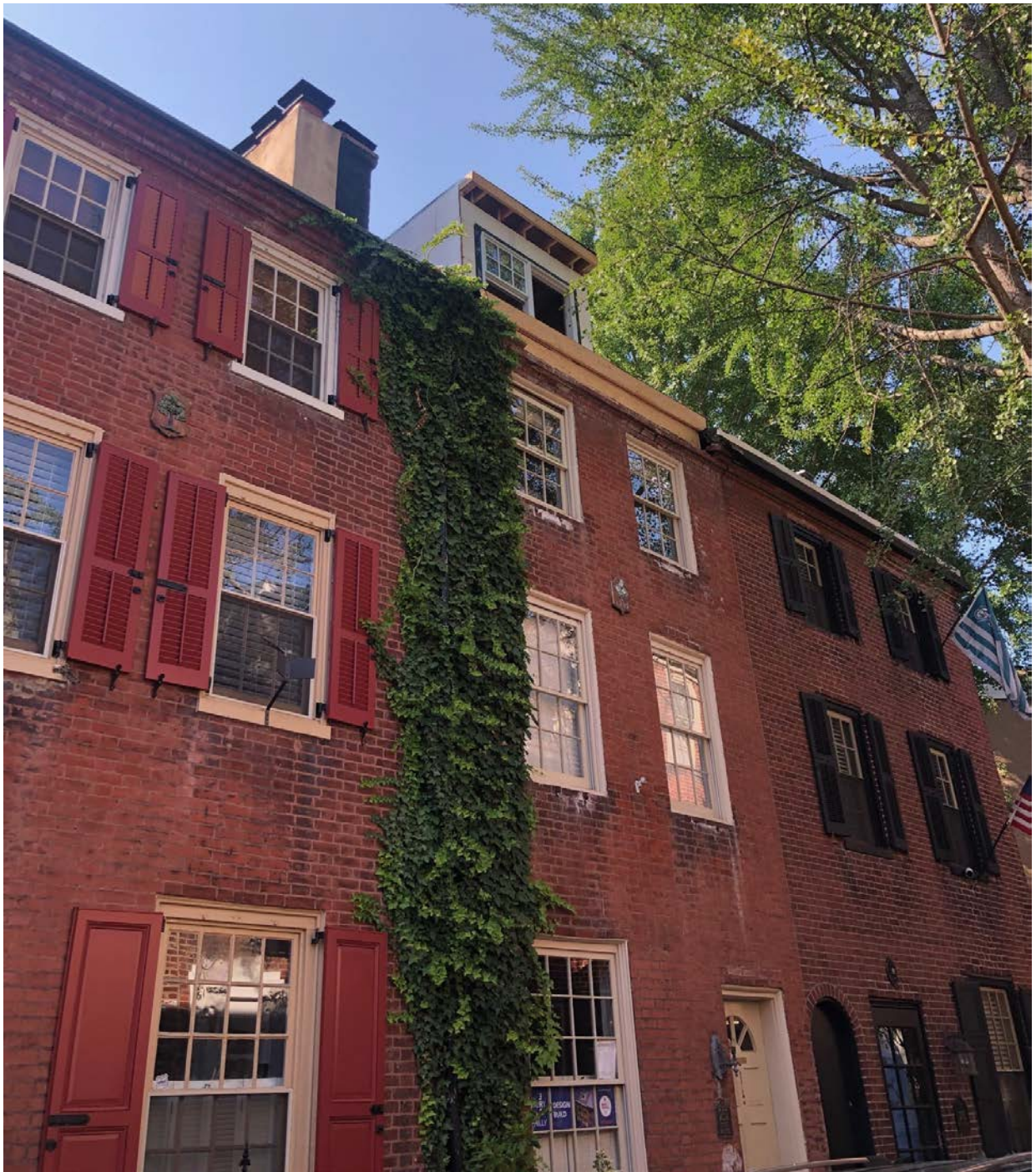
Figure 5: Front façade of 252 Quince Street, August 2024.
