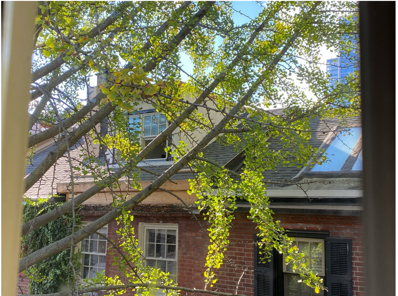
Figure 1: As built condition of front roof, November 2024.
