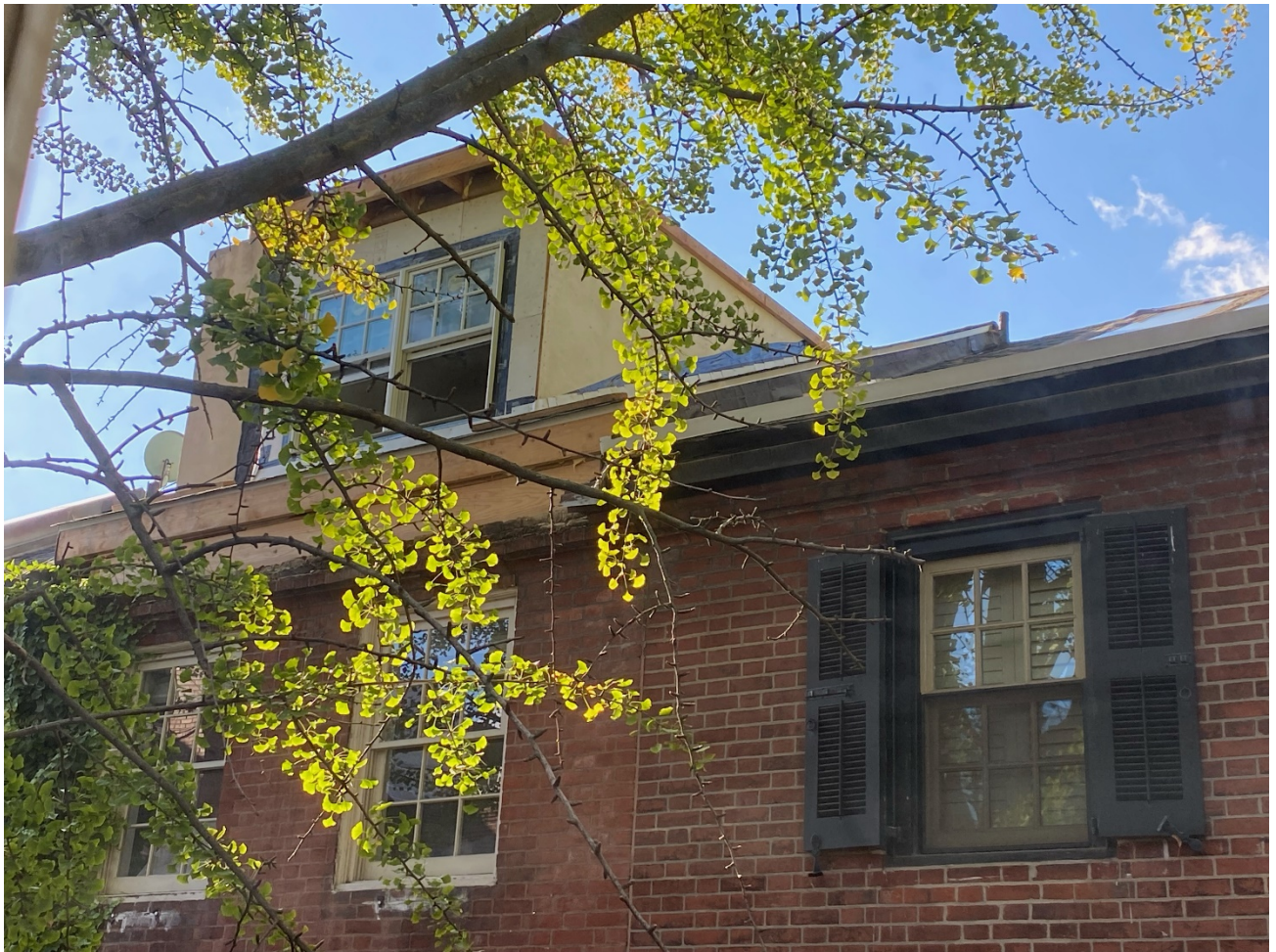
Figure 2: As built condition of front roof, November 2024.
