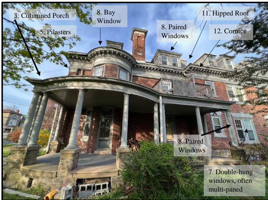
Figure 27. The southwest elevation.
