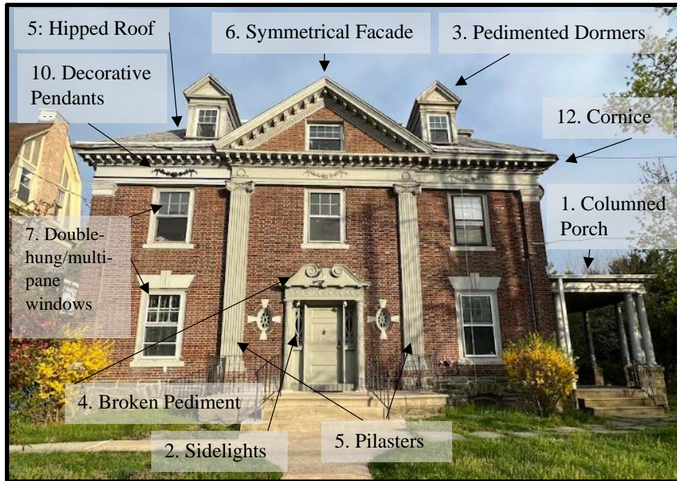
Figure 26. The northwest (primary) elevation. Source: Keeping Society of Philadelphia, 2023.
