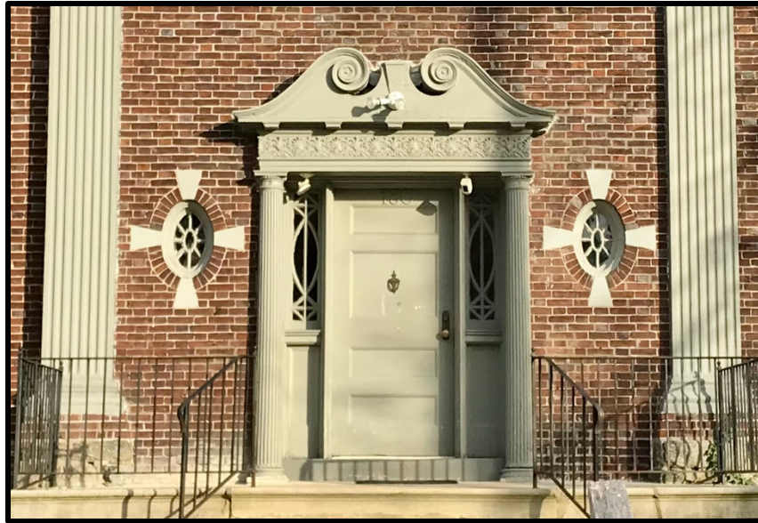
Figure 6. Detail of principal entry door at northwest (primary) elevation. Source: Keeping Society of Philadelphia, 2023.
