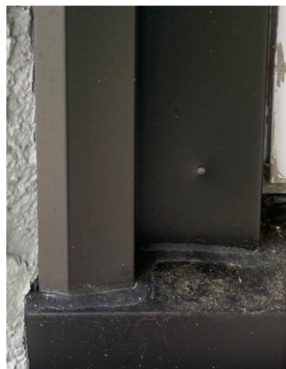
Fig. 6a. Typical window surround and sill, all modern materials
