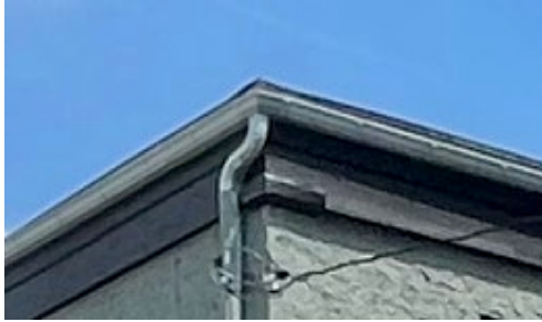
Figs. 4, 4.a. Corner of third floor cornice
