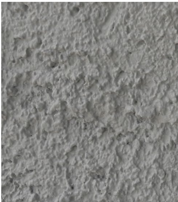
Fig. 9. Gunite surface sprayed on painted, non-historic stucco surface
