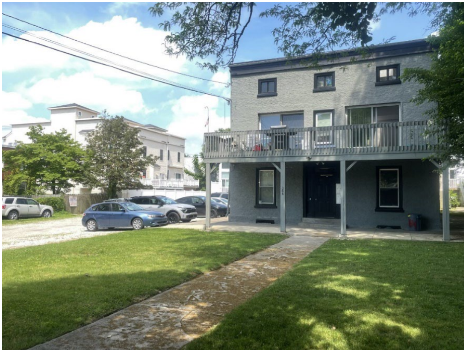
364 Lyceum Avenue, photograph in June, 2024 matching its appearance at the time of the designation. Modern buildings on all sides form its setting
