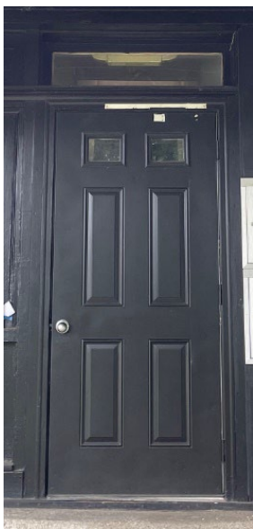
Fig 6. Front Steel Door
