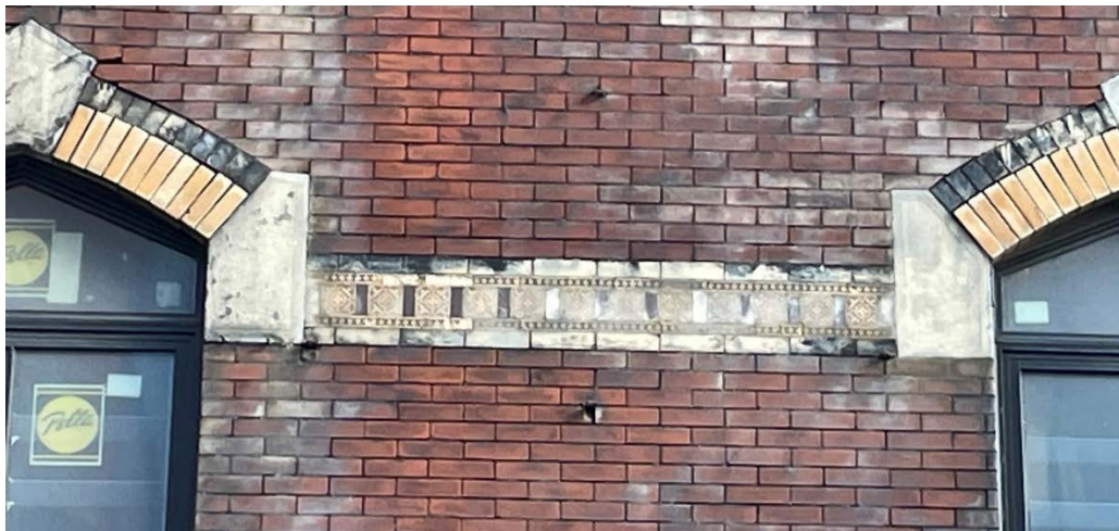
Figure 37: Detail showing decorative band on the second floor.
