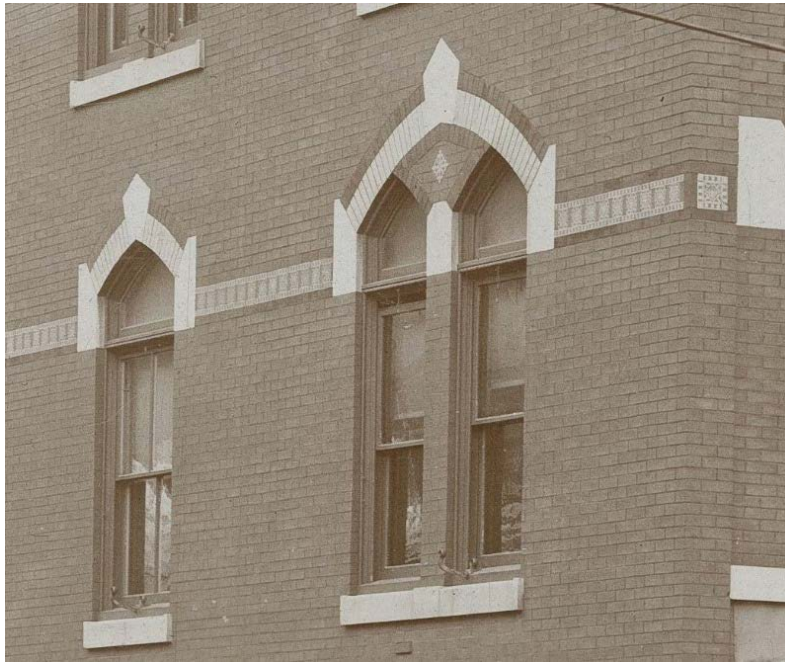
Figure 38: Detail of a turn-of-the-century photo shows the tile before it was painted over, as well as the window arrangement which previously existed on the right-most bay on the 11th Street elevation.
