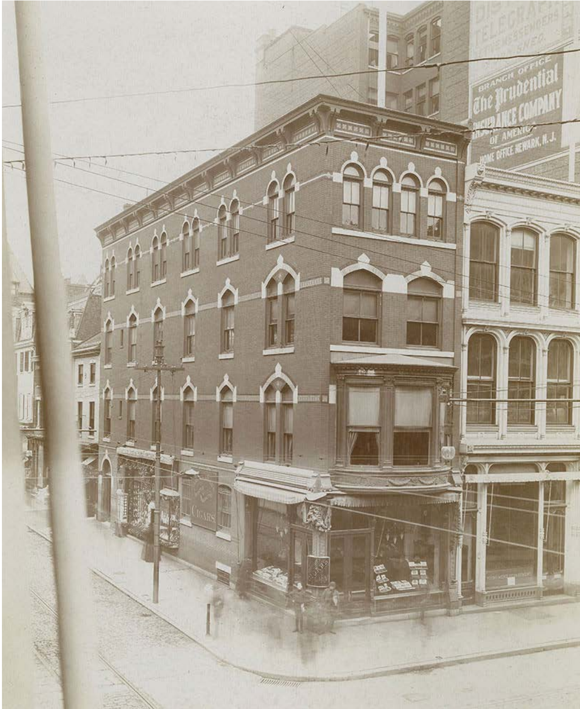
Figure 9: Turn-of-the-century photograph from the Frank Taylor Photographs collection at the Free Library of Philadelphia. The shortening of the building in the early twentieth century led to significant modification of the paired windows along the southern edge of the façade.
