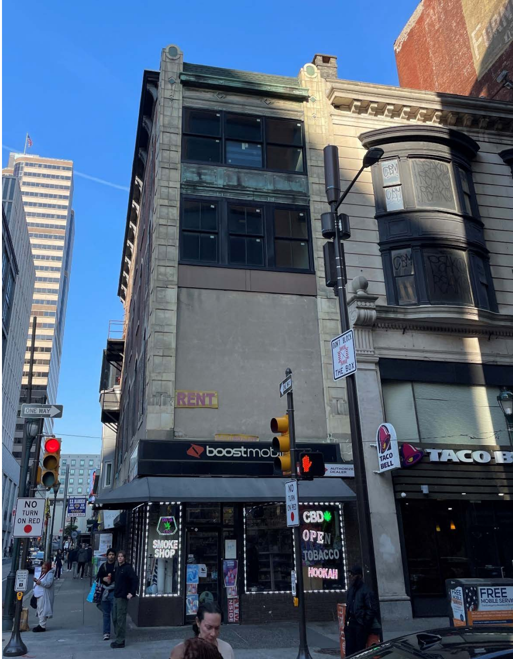
Figure 13: The Chestnut Street elevation features prominent pilasters topped with inverted teardrop ornaments.
