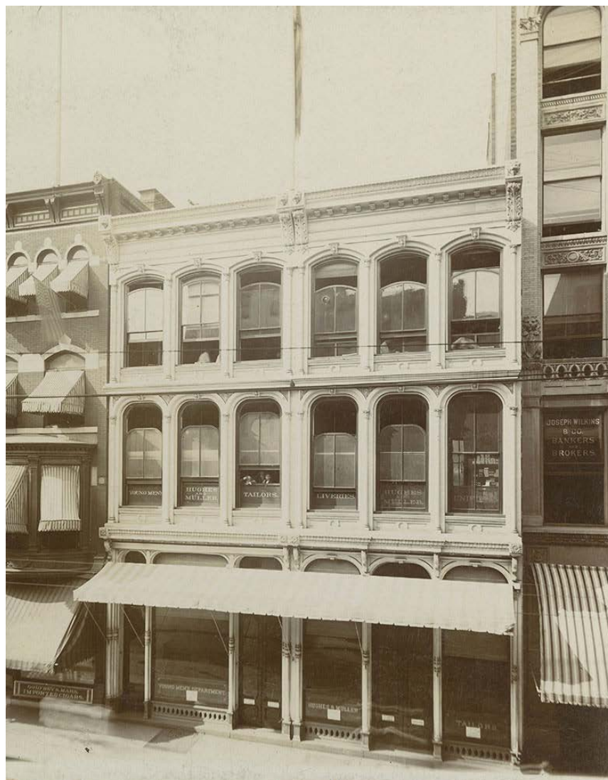
Figure 12: Photograph of 1035-37 Chestnut Street by photographer Frank Taylor shows the awnings extended on 1039 Chestnut Street at left.
