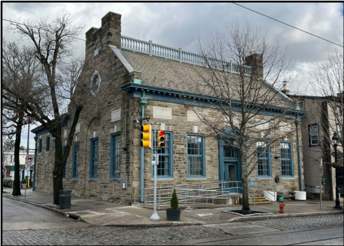
Figure 1. The Chestnut Hill Office of the Germantown Trust Company, 8527-29 Germantown Avenue, Side (Northwest) and Primary (Southwest) Elevations. Source: Oscar Beisert, 2024.
