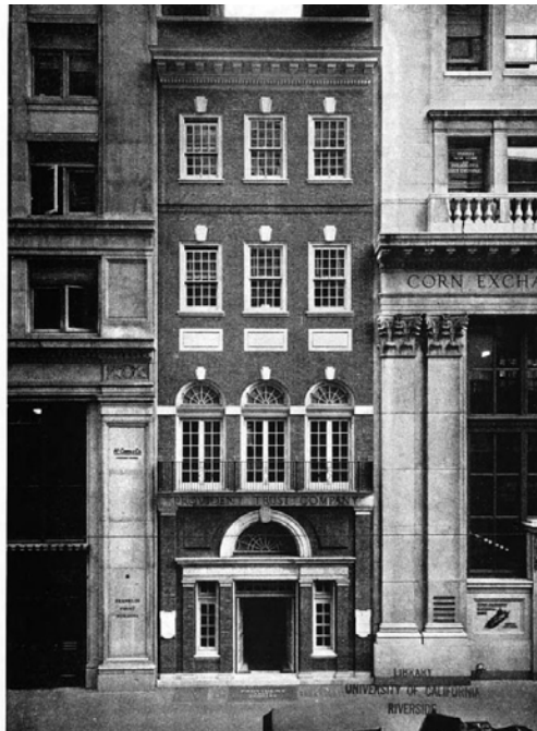
Figure 1 – The Provident Trust Company Building at 1508 Chestnut Street (extant), designed by Carl Ziegler and built in 1925. This image appeared in the July 1925 edition of The Architect .
