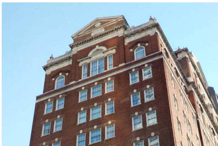
Photo 3 – North elevation, showing the uppermost stories.
