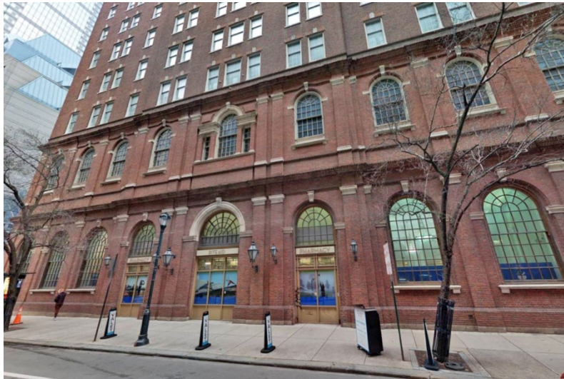
Photo 4 – West elevation, showing the lower stories.
