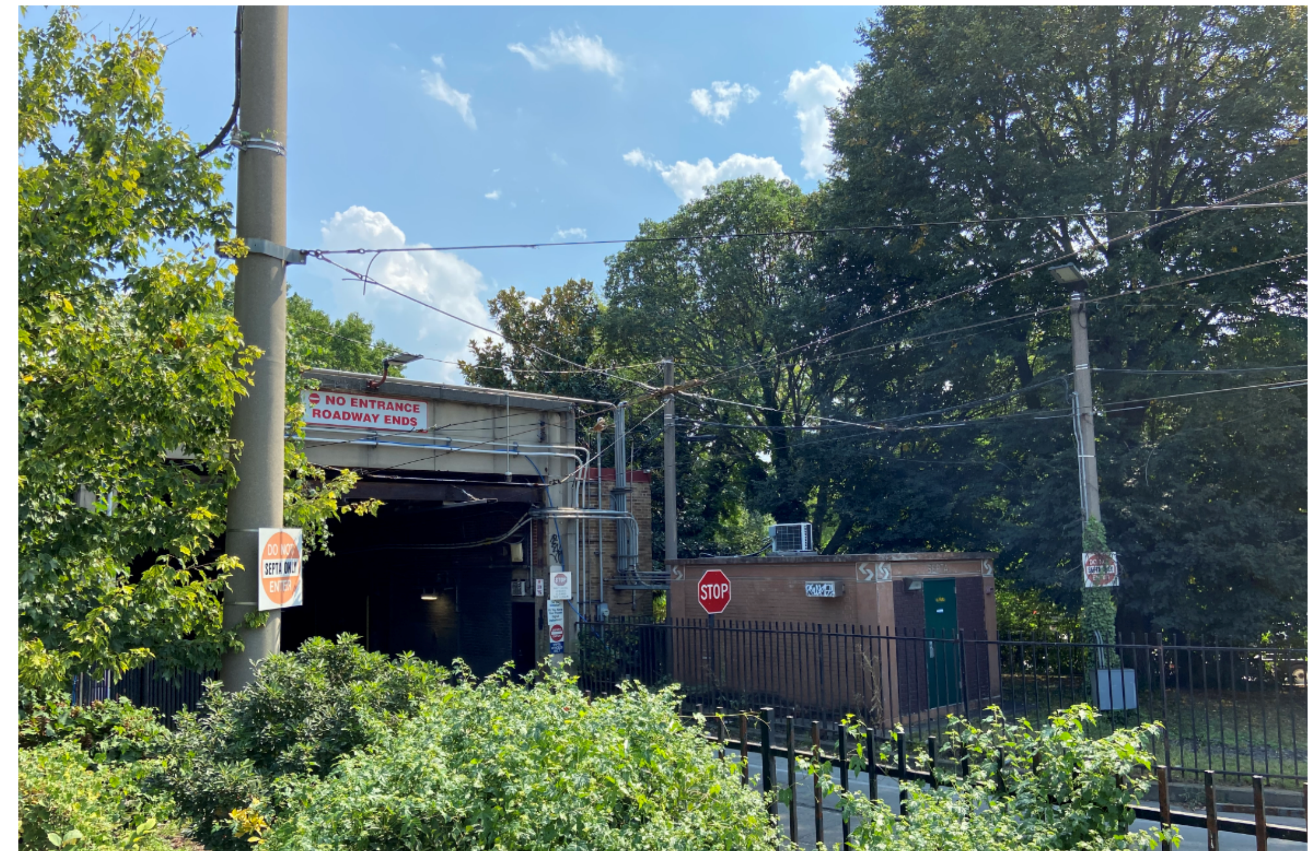
Trolley Portal on West Side of Property - Looking Southwest
