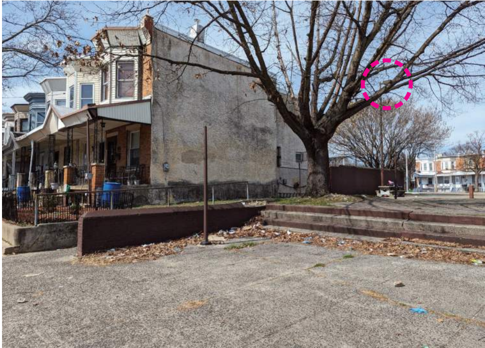
EXISTING POLE LIGHT FIXTURE TO BE REPLACED
