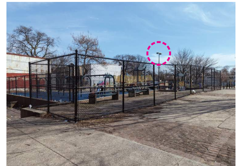
EXISTING POLE LIGHT TO BE REPLACED
