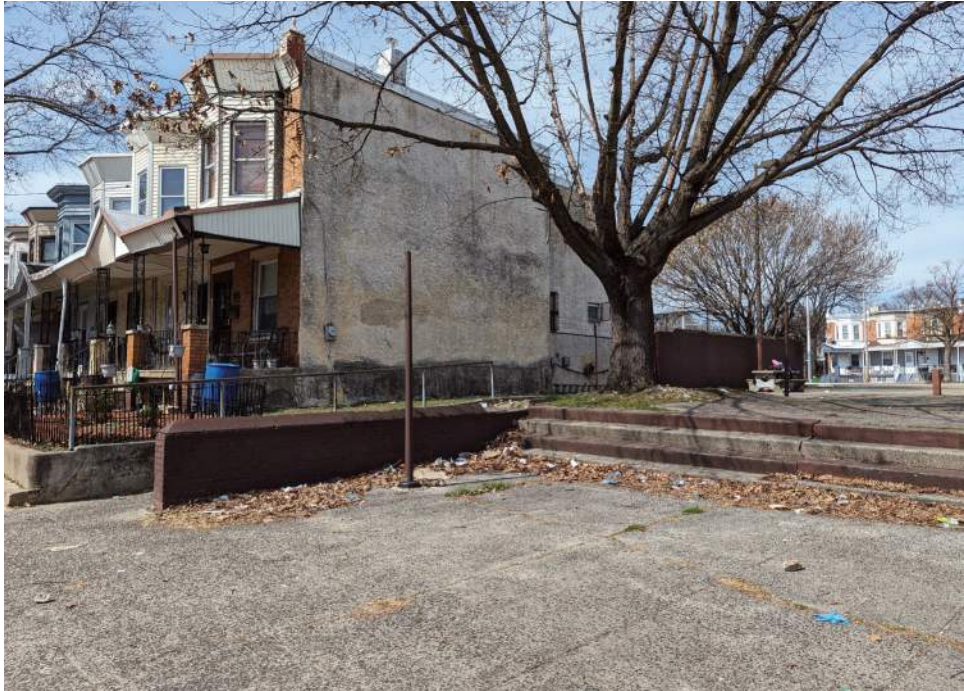
FIGURE 1: NON-COMPLIANT RAMP & TREE IN DECLINE
