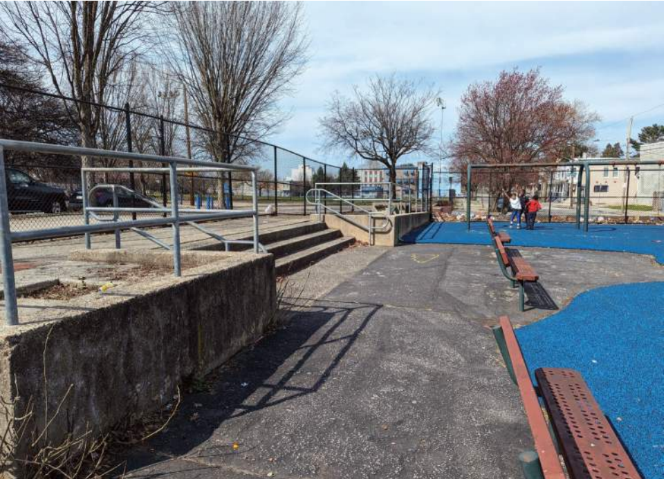
FIGURE 2: WEST ACCESS STAIRS
