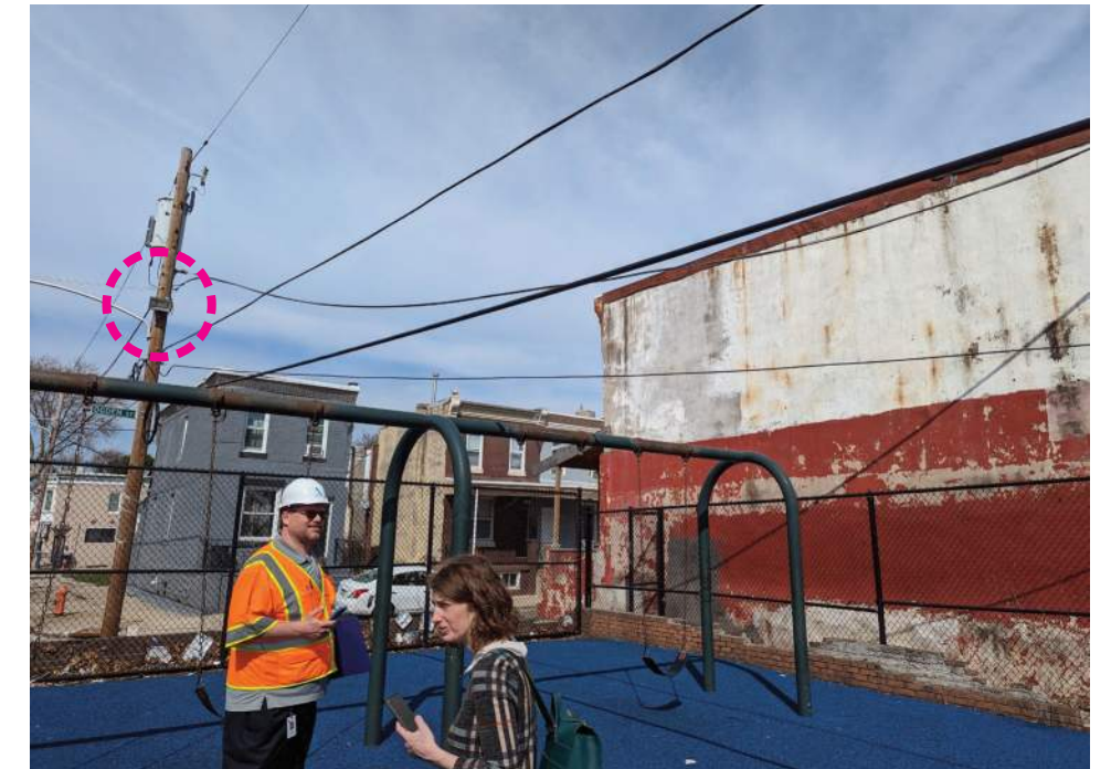
EXISTING FLOOD LIGHT ON UTILITY POLE
