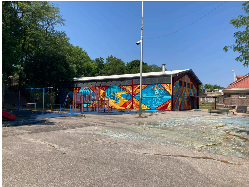
View from SE corner of playground toward gymnasium
