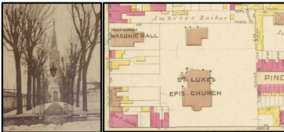
Figure 26. Left: The alley from Germantown Avenue to St. Luke's Episcopal Church at 5409-11 and 5419 Germantown Avenue. Source: GHS. Figure 27. Right: St. Luke's Episcopal Church, as shown on the 1889
