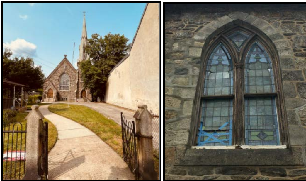
Figure 9. Left: The Gothic Revival gate posts at the street frontage along Germantown Avenue of St. Stephen's M. E. Church. Source: Oscar Beisert, 2023. Figure 10. Right: A typical pointed-arch opening within the original volume of St. Stephen's M. E. Church, featuring stained glass. Source: Aaron Wunsch, 2024.
