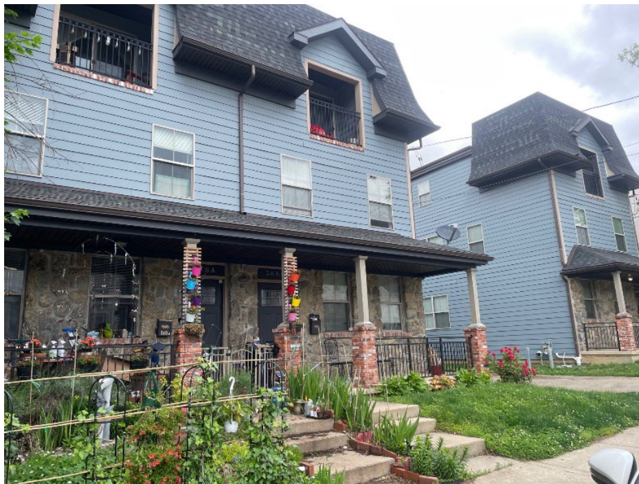
The adjacent houses at 368 a. & b (left). and 368 c (right) were built to the east of 360 -66 in 2012 (permit).
