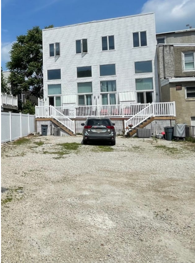
Modern materials and window types and rear entrances onto parking lot at rear of 353-355 Conarroe Street looking NW.
