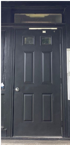
Fig 6. Front Steel Door
