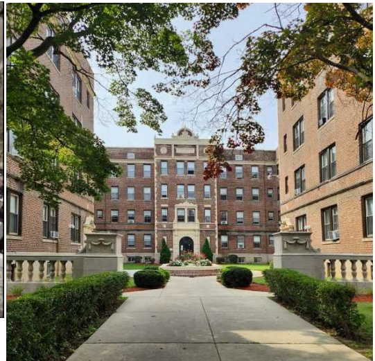
Entry Courtyard View: Cynthia Dutwin
