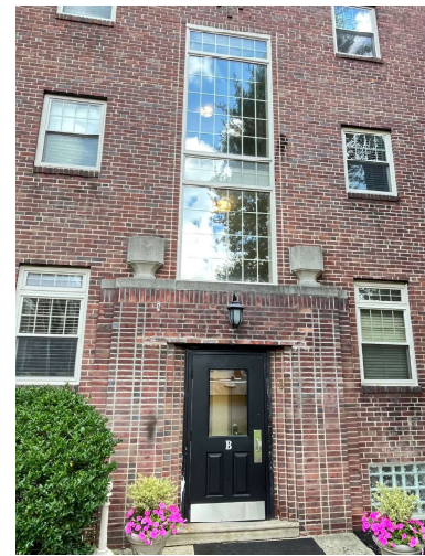
Detail Building A image: Douglas Kingsbury
