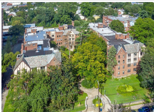
Aerial View: google maps
