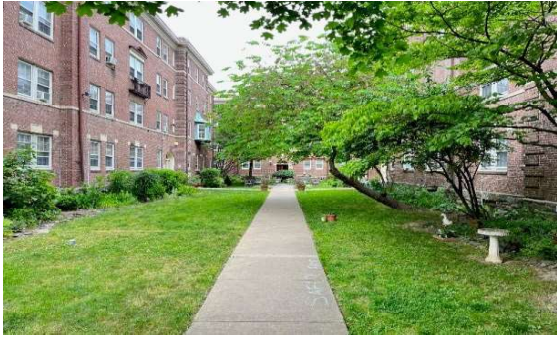
Courtyard View, Looking North Image: Douglas Kingsbury
