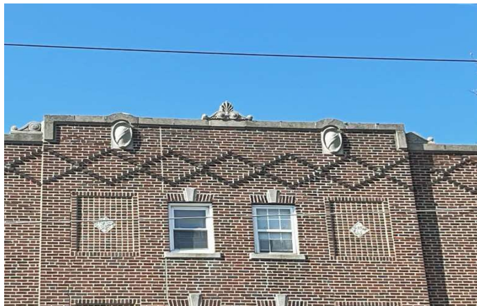
Rear Stair Towers: Libbie Hawes
