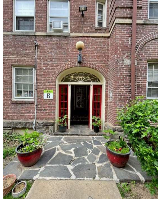
Typical Entry Detail View Image: Douglas Kingsbury
