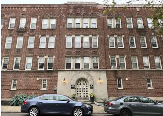
Northwest Facade View: Douglas Kingsbury
