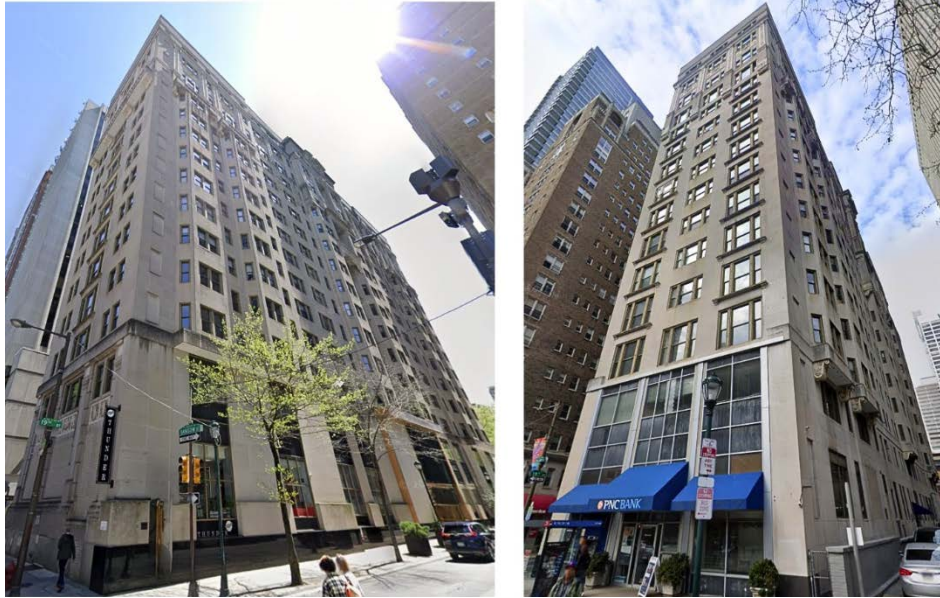
Figure 23. The Wellington apartment building. Images courtesy of Google Maps.
