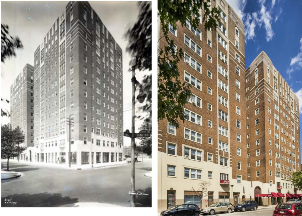
Figure 25. Garden Court Plaza apartment building. The left image is courtesy of the Philadelphia YIMBY blog and the right image is courtesy of the Mid Atlantic Real Estate Journal.
