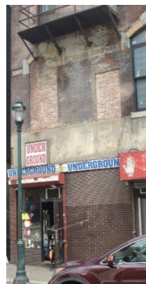
Present condition: shop front
