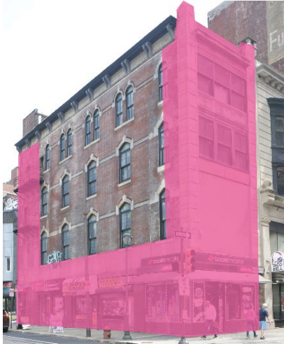
Altered or removed original fabric on both facades
