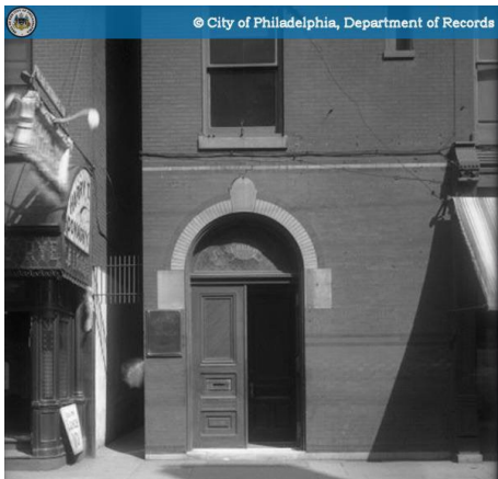
Original doors on 11 th Street to upper level, 1912
