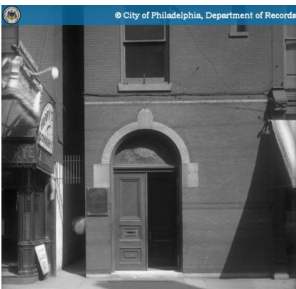
Original doors on 11 th Street to upper level, 1912
