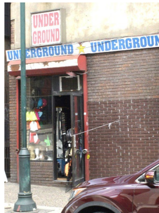
Present shop front in place of door: no door to upper levels
