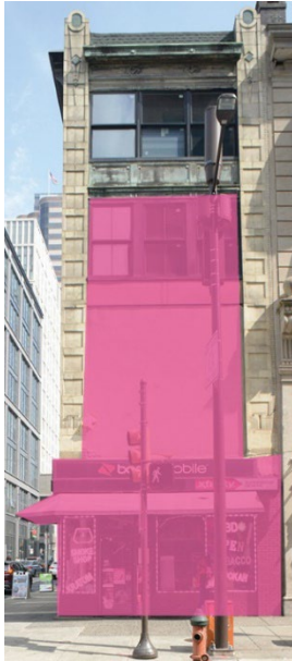
2024: 1st and 2 nd floor facades removed
