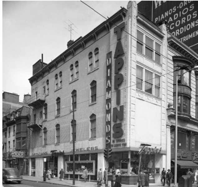
Pre-1952: brick painted, 2 nd floor elements removed and 1 st floor redesigned (Athenaeum, George Thomas donation, Stelman Collection)
