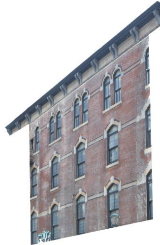
What remains of the 1870s building
