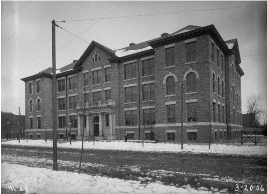
1906 view of Abigail Vare Elementary School, Morris & East Moyamensing Street; James Gaw, architect (The school was named for mother of notorious William Scott Vare who was so corrupt that he could not be seated in US Senate). The building survives in good condition today.
