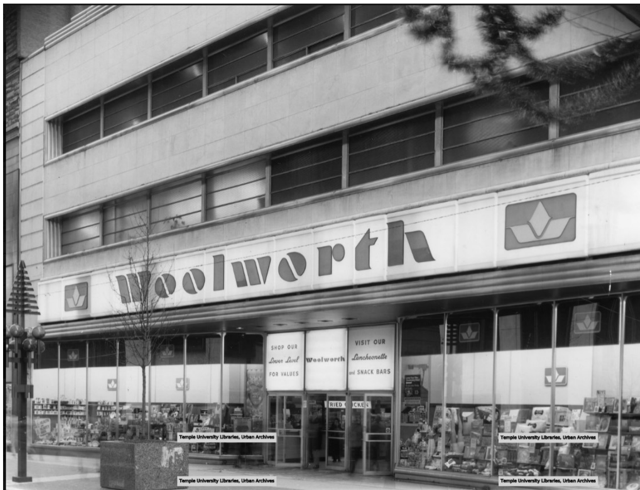
Figure 13. Woolworth store with panel sign, 1979. Source: Temple University Urban Archive.
