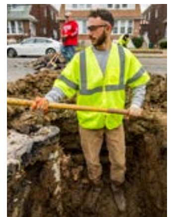
Above: A plumber replaces a service line
