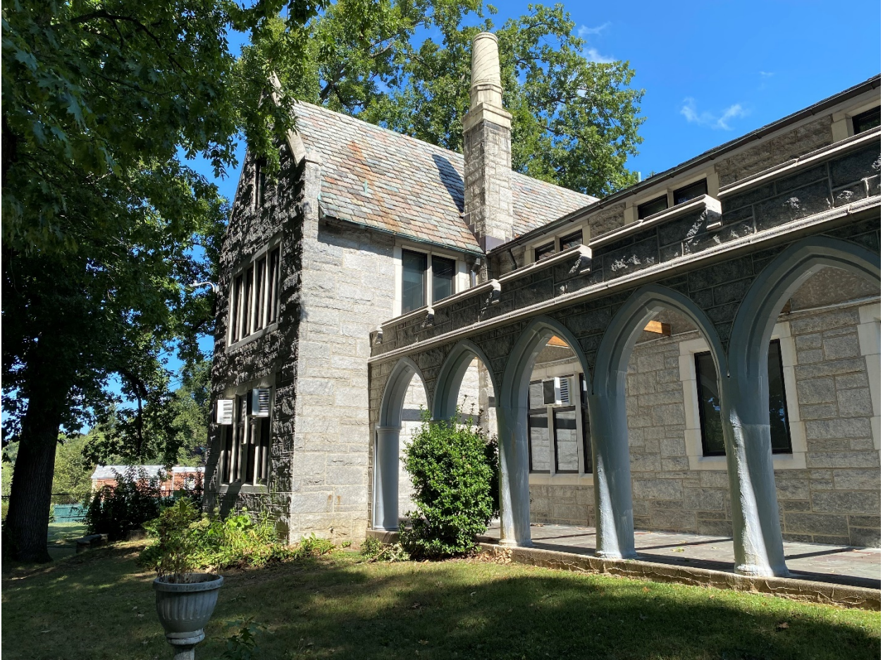
Figure 5. South façade (facing Ardleigh Street), view 1 of 2. Source: Nominator.
