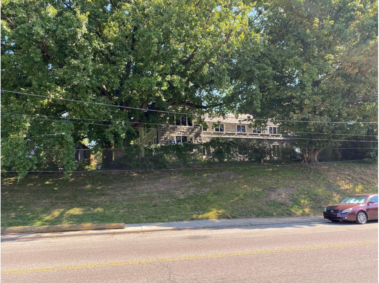
Figure 4. View looking north from Ardleigh Street. Source: Nominator.
