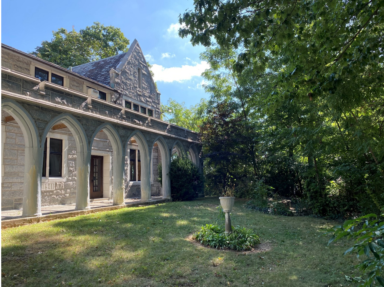
Figure 6. South façade (facing Ardleigh Street), view 2 of 2. Source: Nominator.
