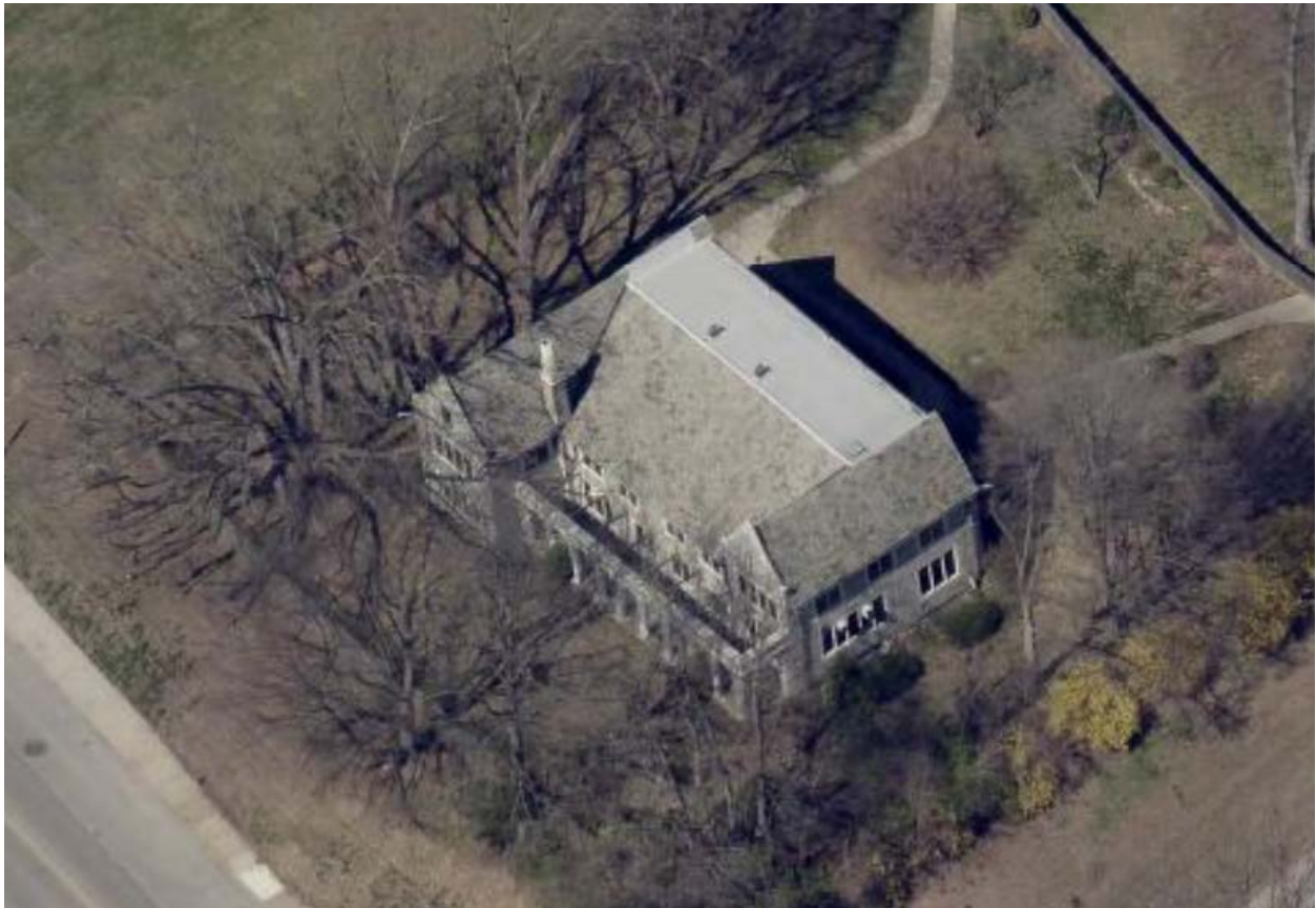
Figure 3. Aerial view of 6633 Ardleigh Street, looking north. Source: Pictometry.
