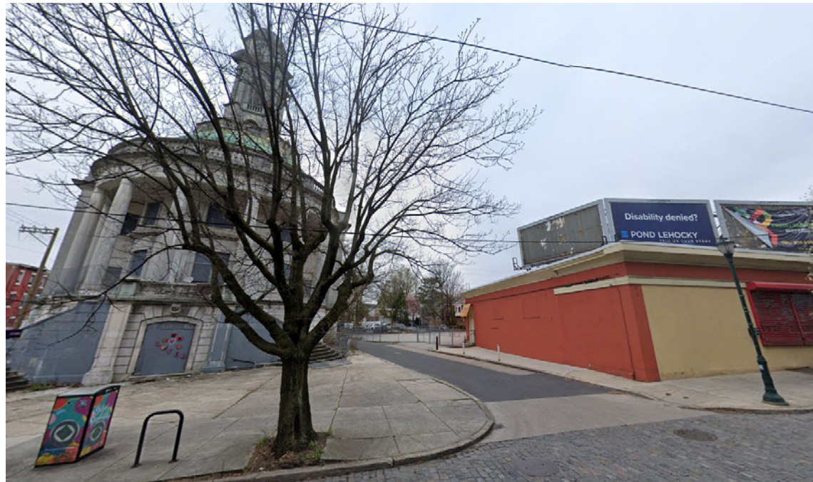
B GERMANTOWN AVENUE LOOKING SOUTH-WEST
