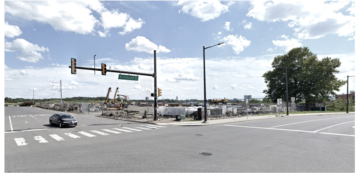
VIEW LOOKING S AT SCHIRRA + RICHMOND
