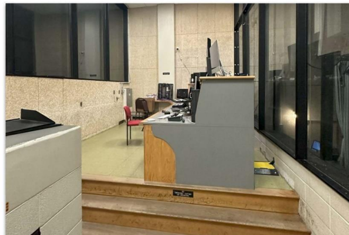
OUTDATED AND INACCESSIBLE STUDIO CONTROL SPACES WITH LACK OF ACOUSTIC CONTROL
