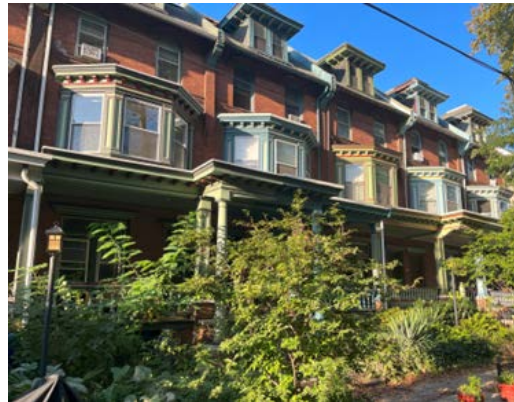
Figure 18. 4200 block of Osage Avenue, view to northeast. This block represents a typical late 19 th c. development type.
