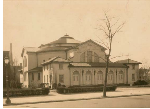
Figure 21. Former First Church of Christ Scientist, 4017 Walnut Street, exterior view, c. 1915. (The University of Pennsylvania Almanac, https://almanac.upenn.edu/archive/volumes/v57/n32/rotunda.html .)
