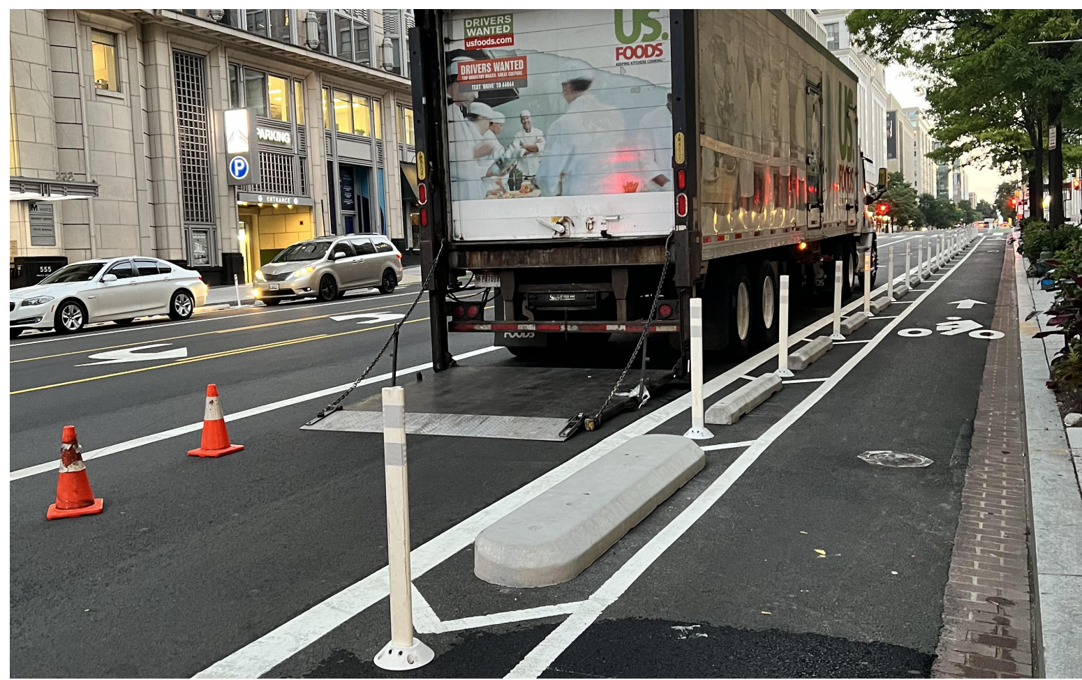
Example of concrete curb sections separating a bike lane in Chicago
