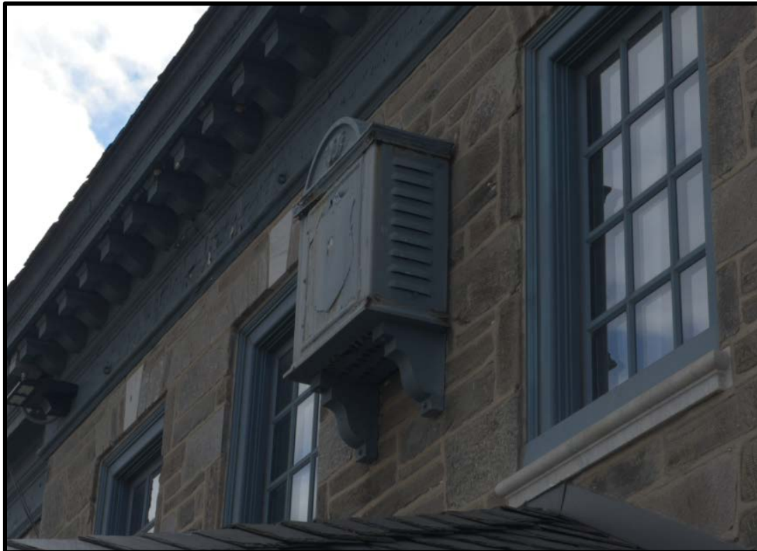
Figure 10. An early alarm device on the Chestnut Hill Office of the Germantown Trust Company, 8527-29 Germantown Avenue, Rear (Northeast) Elevation. Source: Oscar Beisert, 2024.
