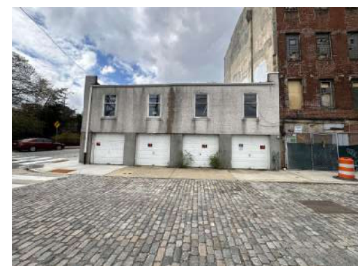
IMAGE 9 - (2024) VIEW OF N. WATER STREET FACADES
