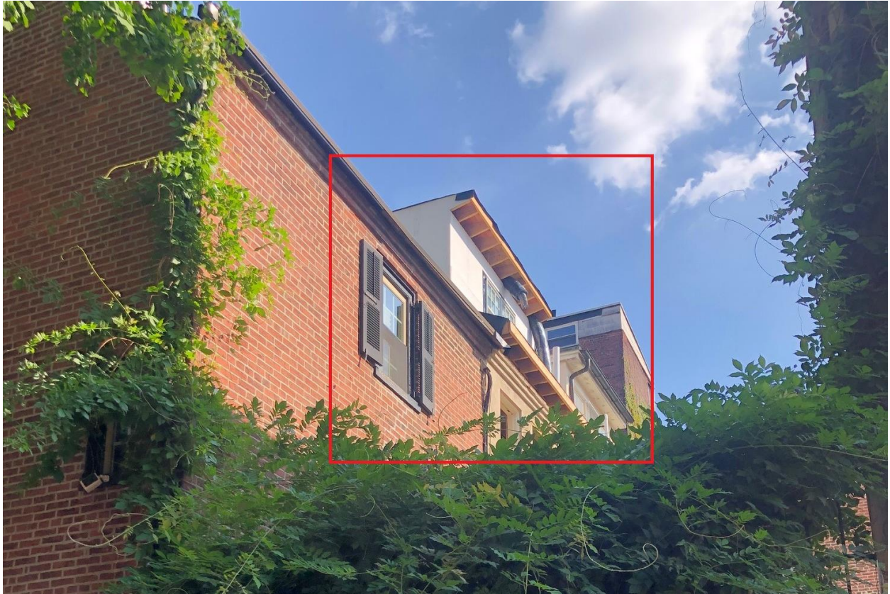
Figure 7: Rear façade of 252 Quince Street as viewed from Manning Street, August 2024.
