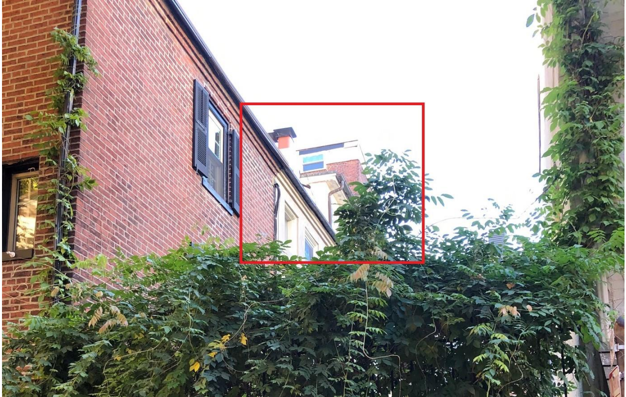
Figure 6: Rear façade of 252 Quince Street as viewed from Manning Street, December 2023.
