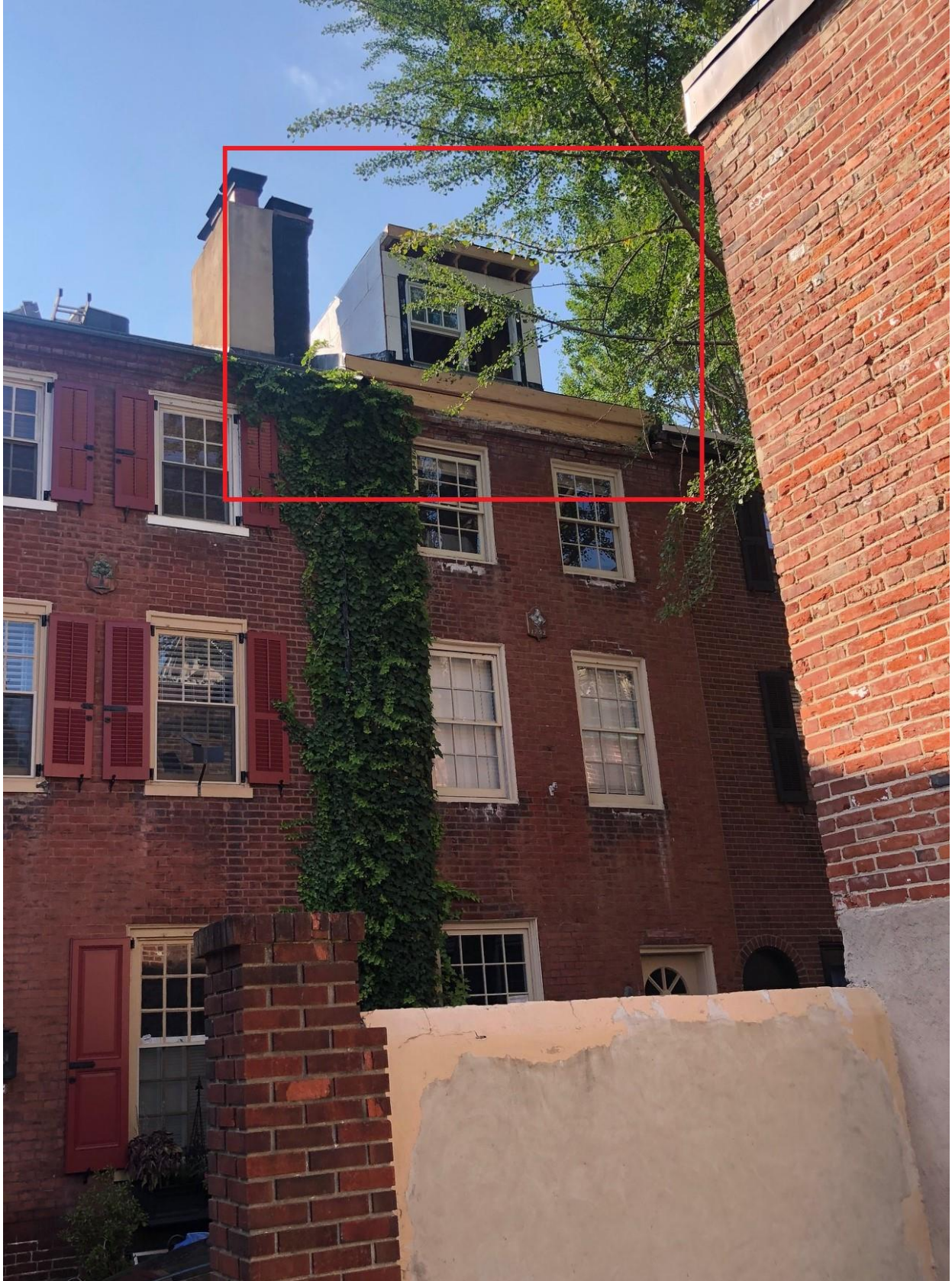
Figure 5: Front façade of 252 Quince Street, August 2024.
