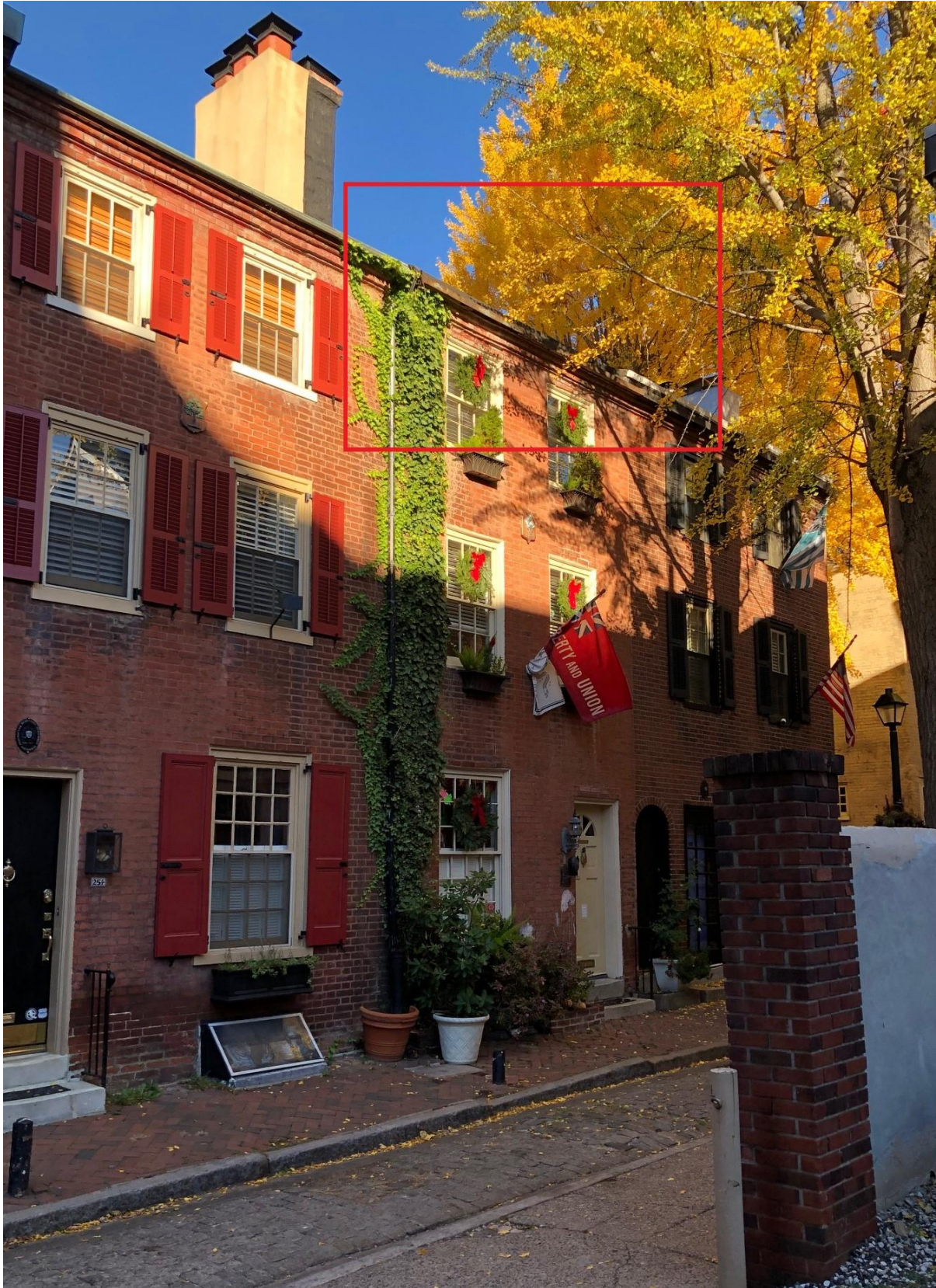
Figure 4: Front façade of 252 Quince Street, December 2023.
