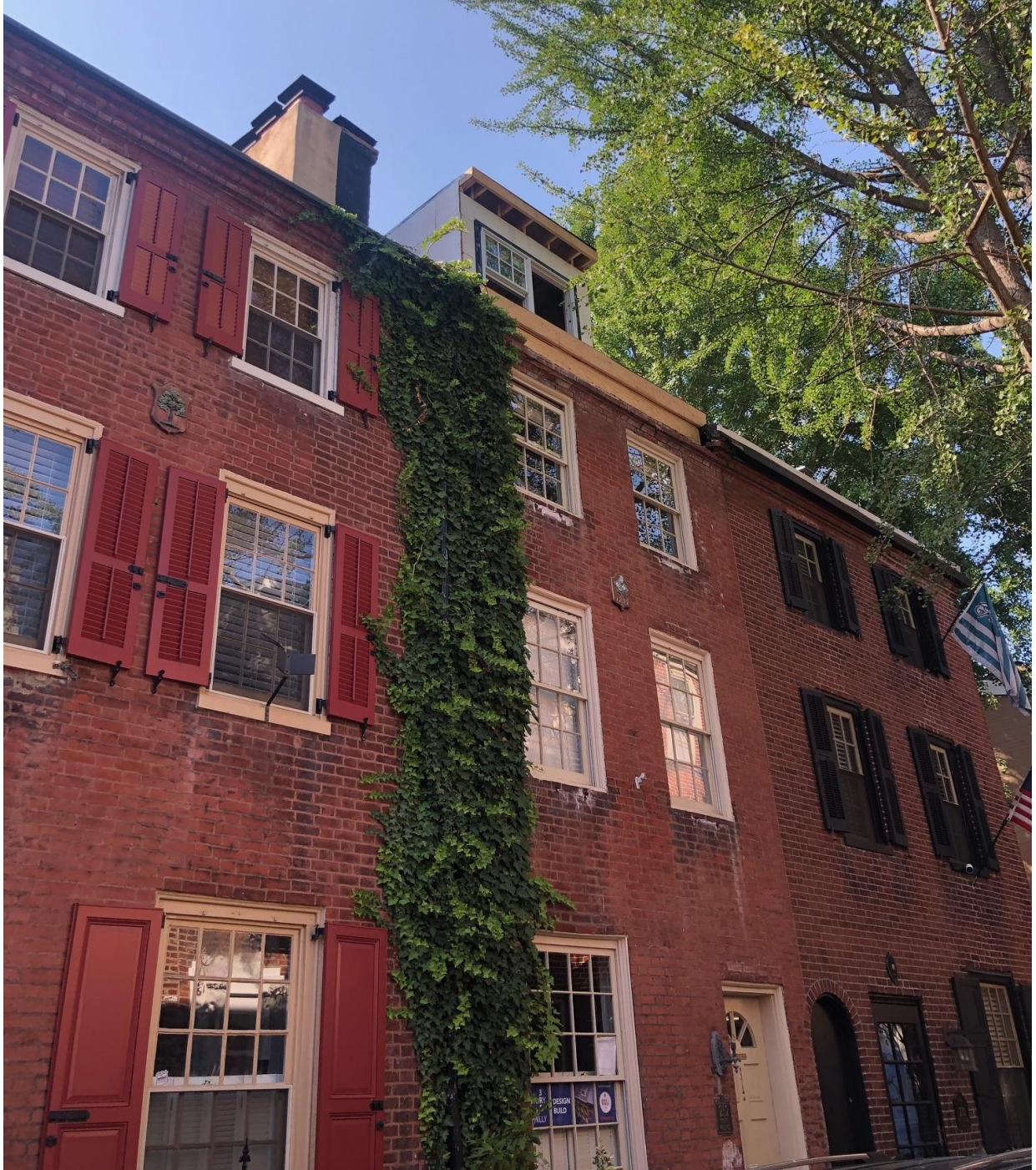
Figure 3: Front façade of 252 Quince Street, August 2024.
