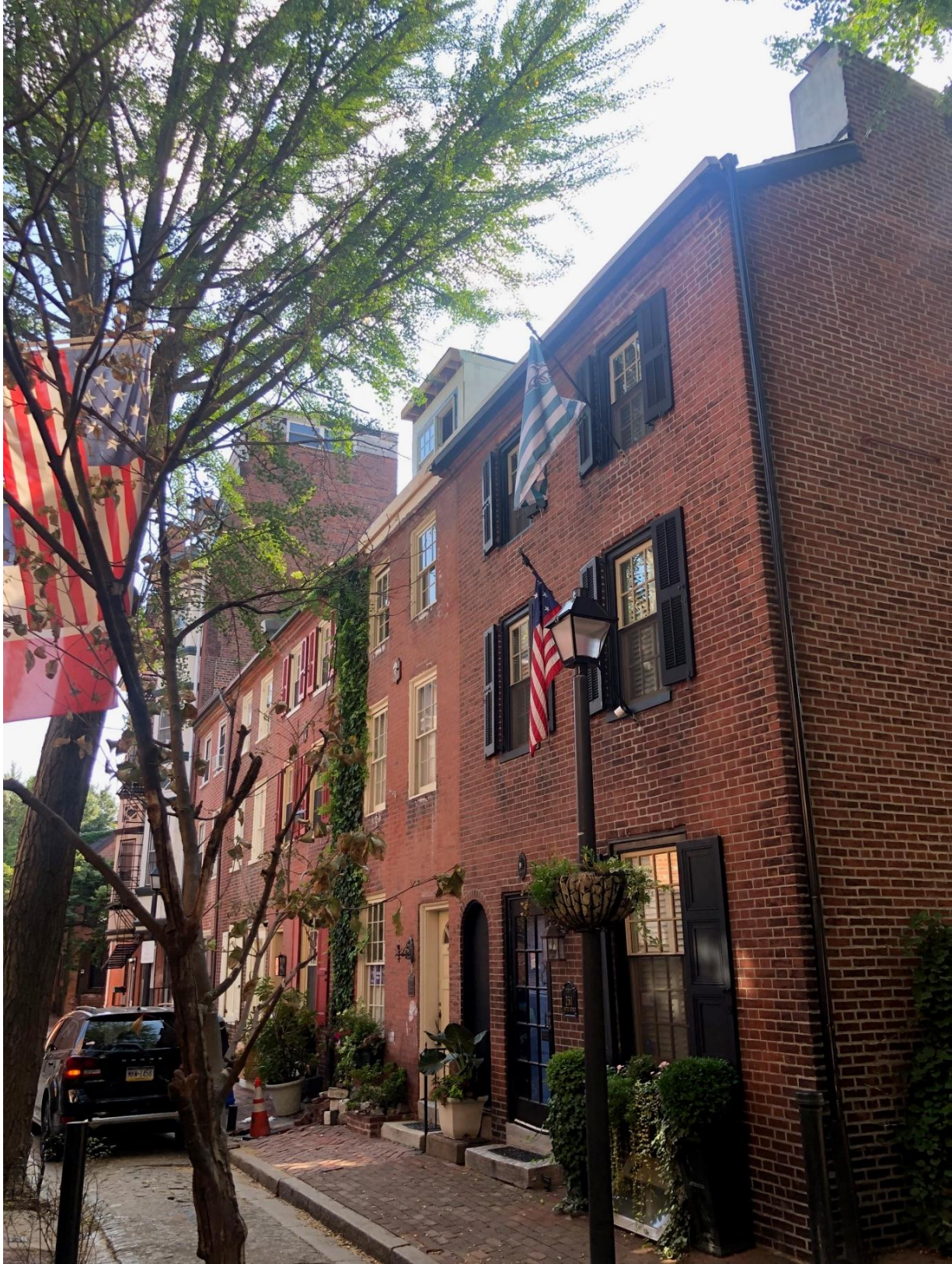
Figure 2: 200 Block of Quince Street in August 2024 while under construction. 250- 258 252 Quince Street is second from right in the image.
