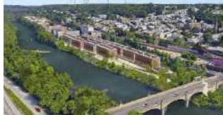
The Locks Riverside Way (1 Leverington Avenue), Philadelphia 5 Stories - 63 Townhomes
