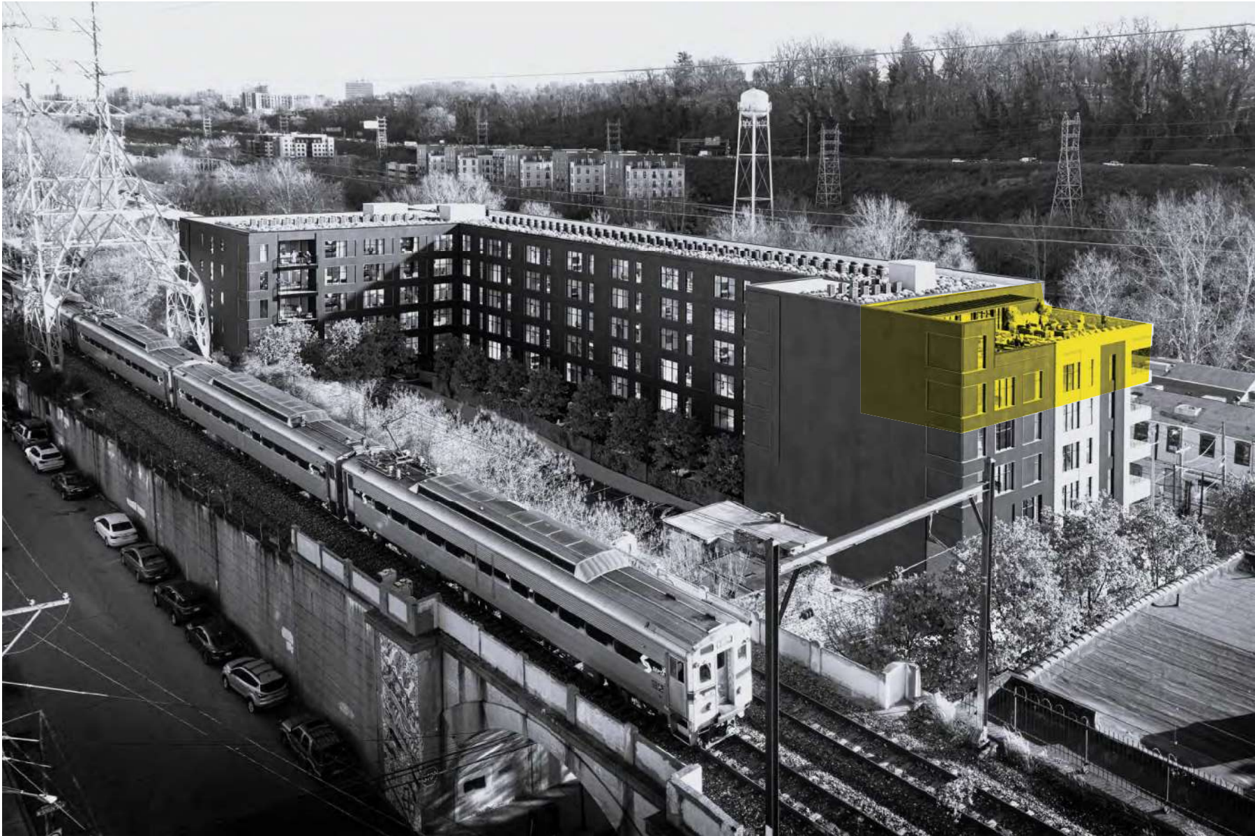
Aerial View looking Southeast - Previous Scheme (May 10)
