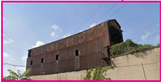
Corrugated Metal Siding at Nearby Rail Spur
